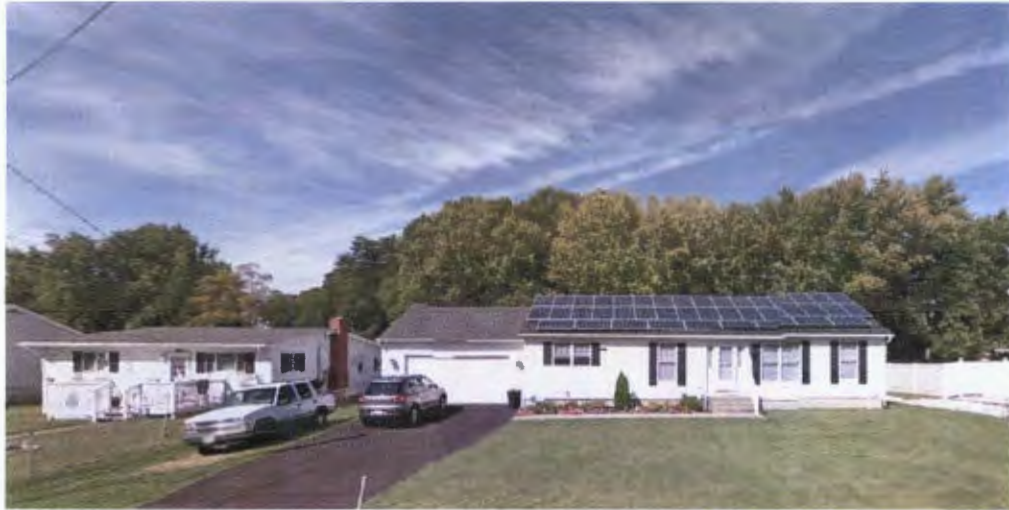
DWELLING ON RIGHT (2414 LODGE FARM RD)
