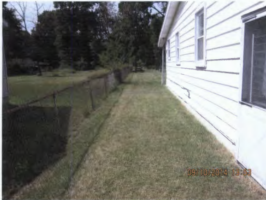
LEFT SIDE LOOKING TOWARD REAR
