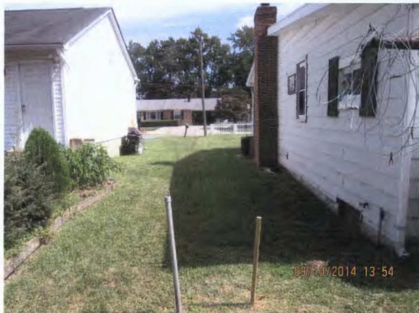
RIGHT SIDE LOOKING TOWARD STREET
