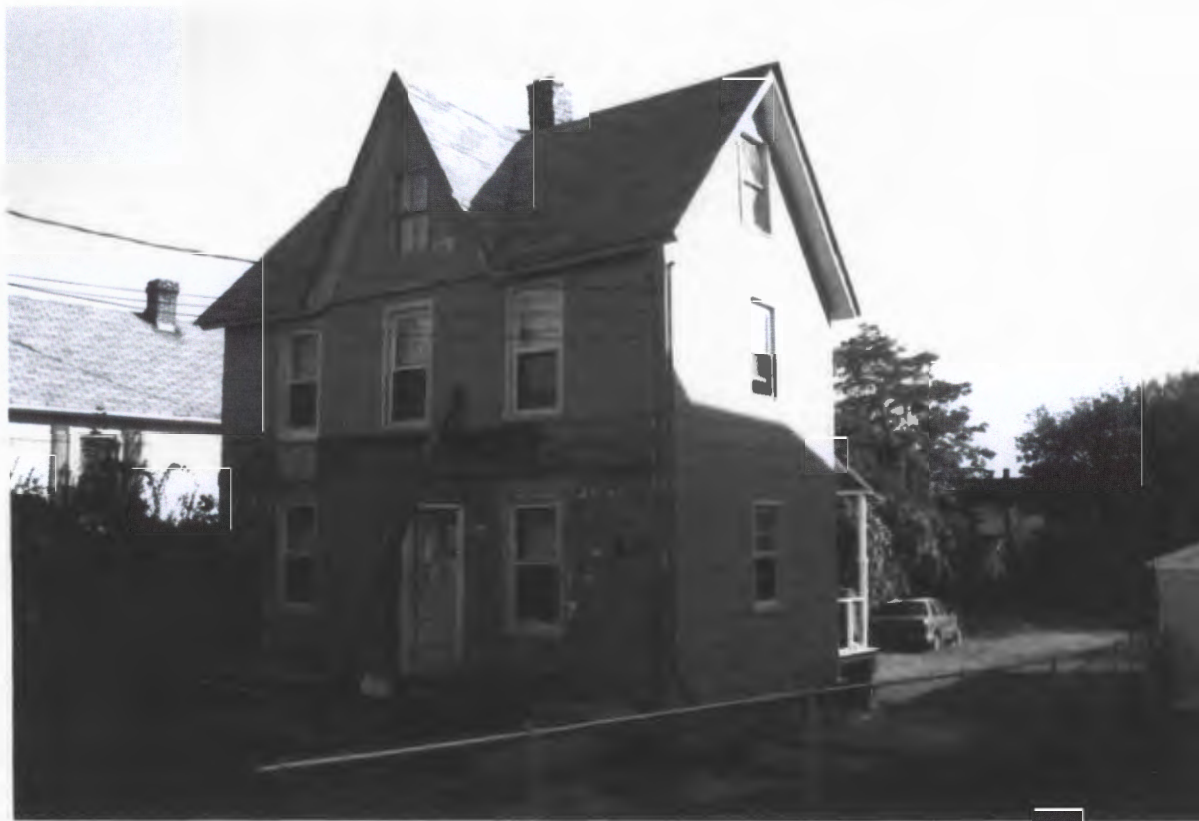
320 Pennsylvania Ave - October 2001
