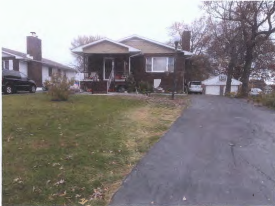
UPPERLANDING RD/ FRONT OF DWELLING
