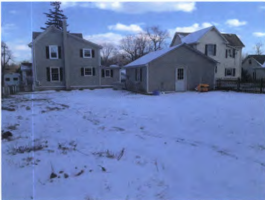
Rear Of 1440 Burton Ave.
