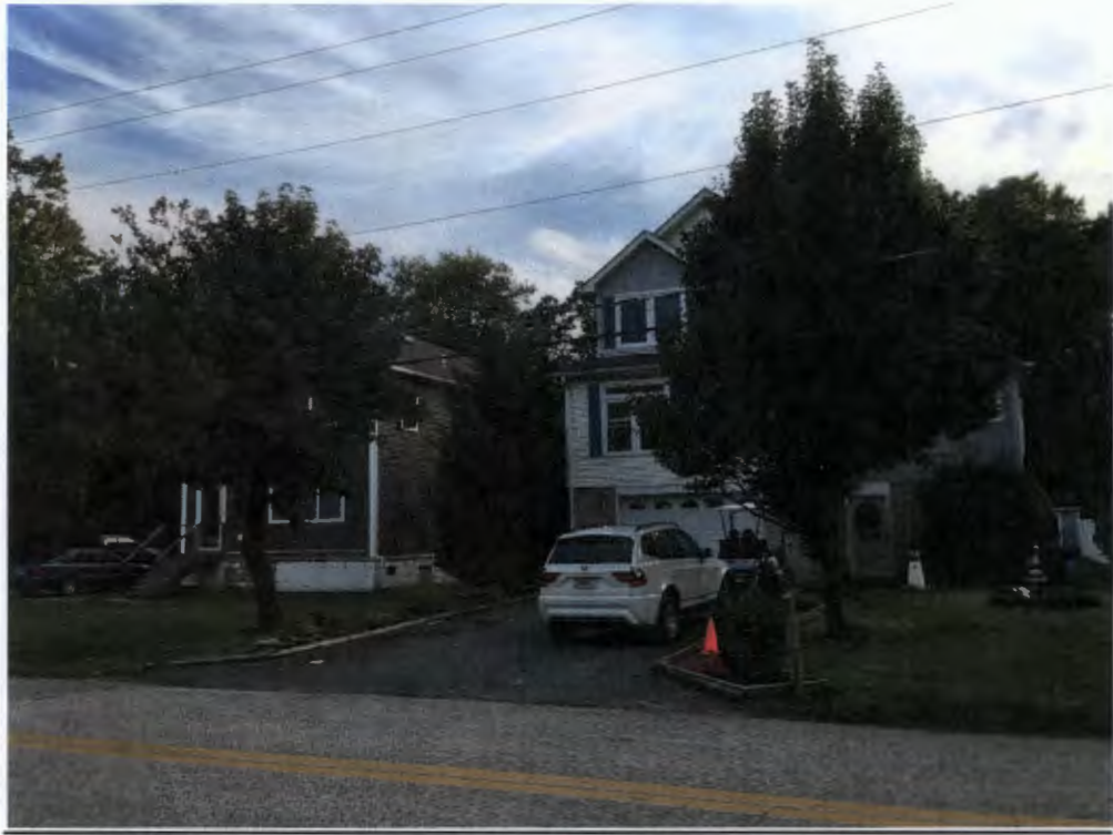
Front view of 8909 Millers Island Blvd.
