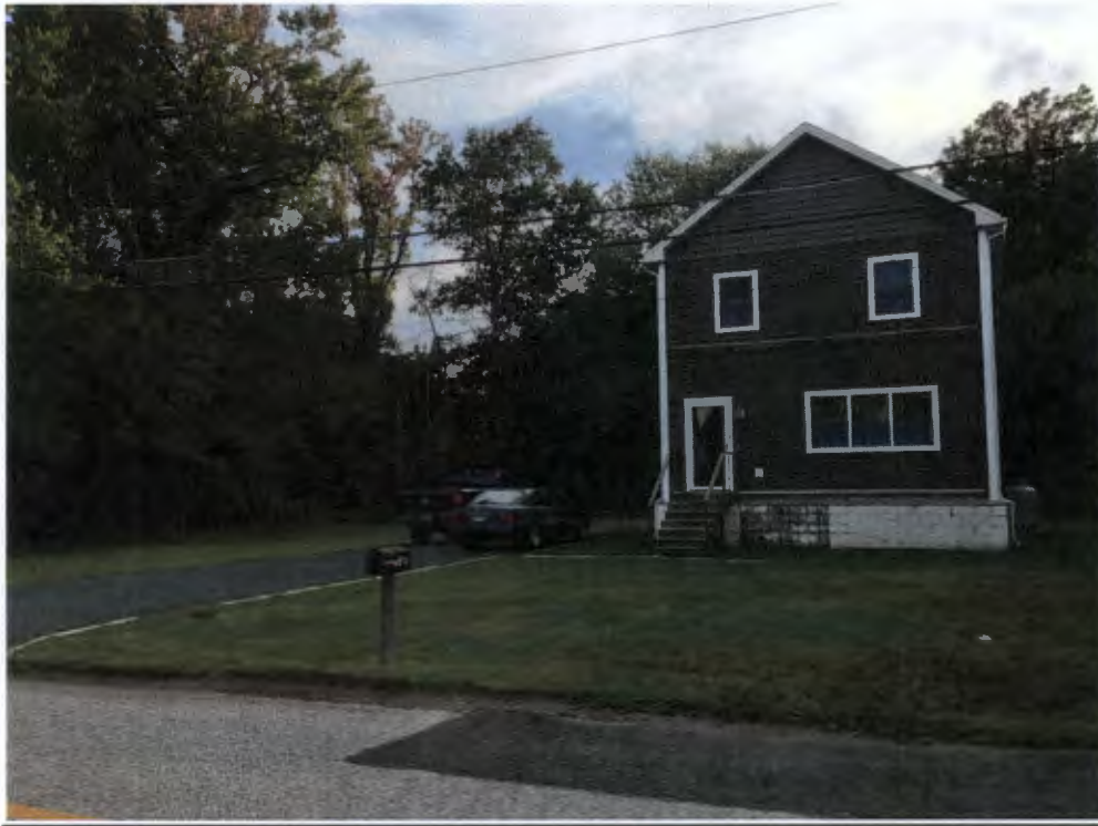
Front view of 8911 Millers Island Blvd.
