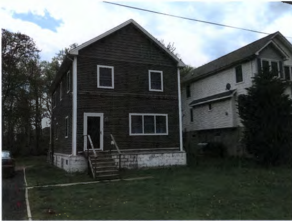
Front view of 8911 Millers Island Blvd. with neighboring residence (8909)
