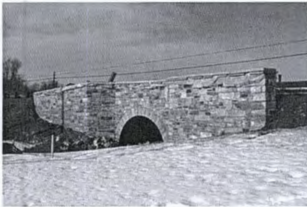
This recently reconstructed bridge over Meadow Run illustrates how small structures similar in scale and proportion to an older structure can be designed to maintain the character of the roadway. In this case some original materials were reused. These are photos of the same bridge, one from the side, looking up and one from the road level view.
