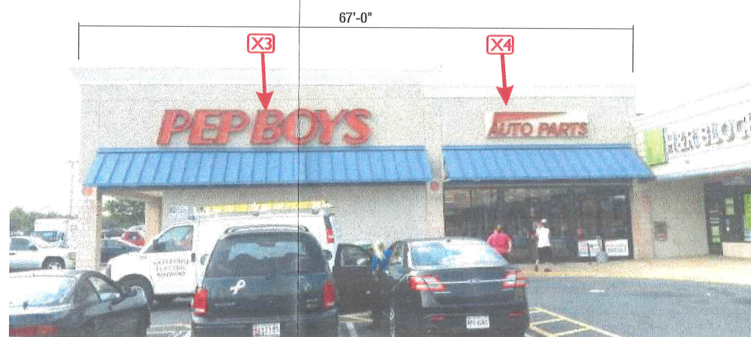
Existing Condition - Right Side Elevation
