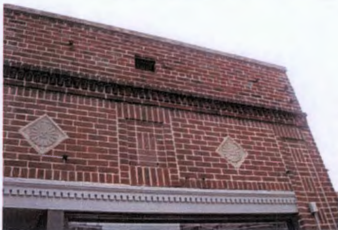
The manner in which stretchers (the long side of the brick) and headers (the ends of the brick) are used, how the rows are laid, and the width, profile and color of the mortar joints, all contribute to the character of brick walls and foundations.
