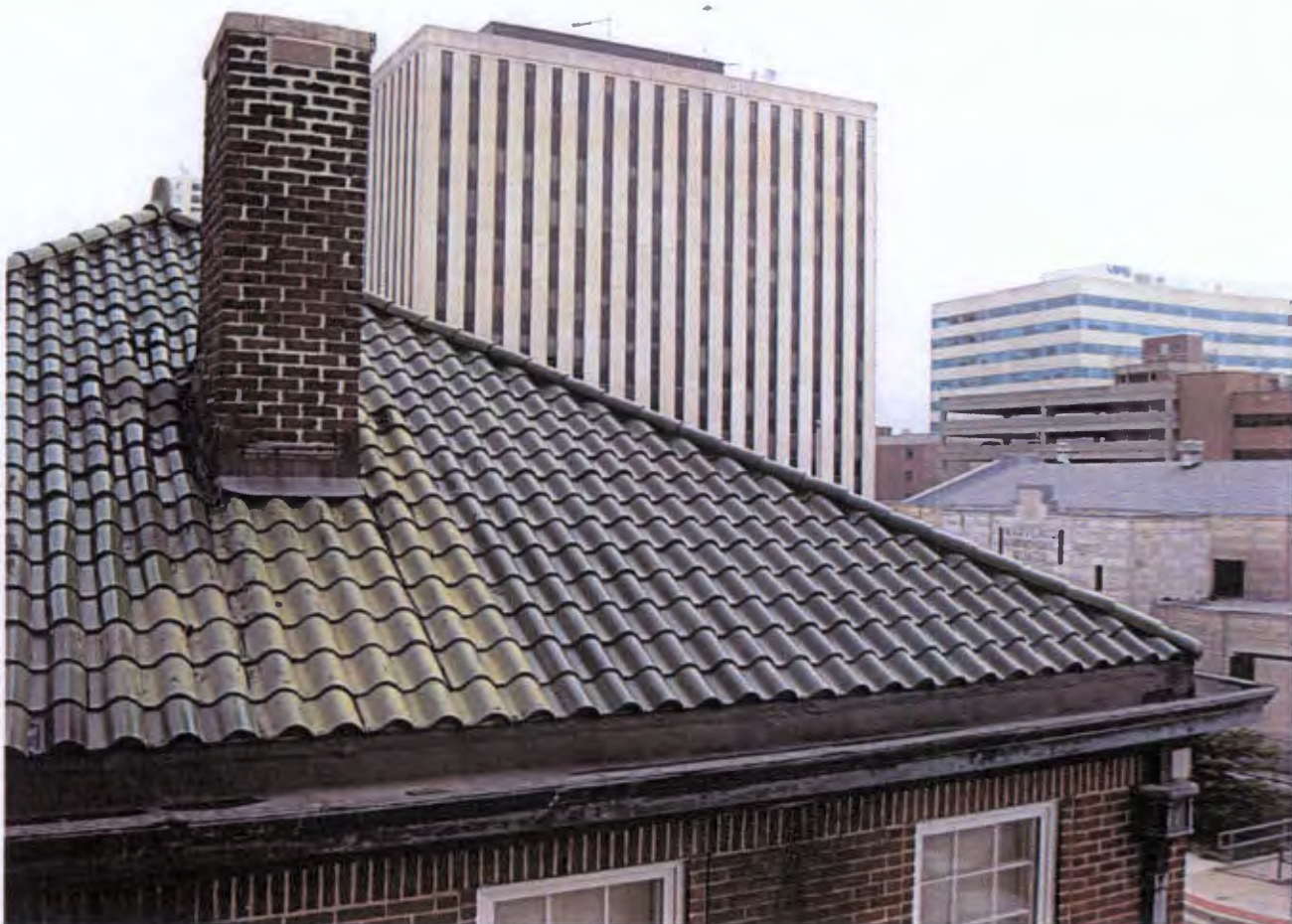
Gutters and downspouts contribute to a roof's character.
