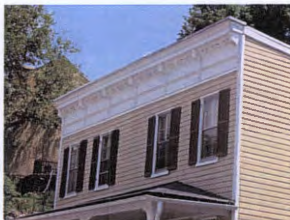
Cornices employ different details such as brackets, modillions and dentils.
