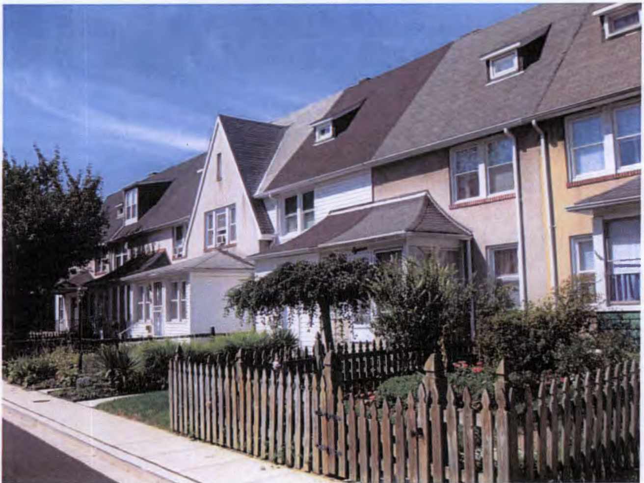
The front porches in this historic community have all been enclosed, which greatly undermines the integrity of the homes.
