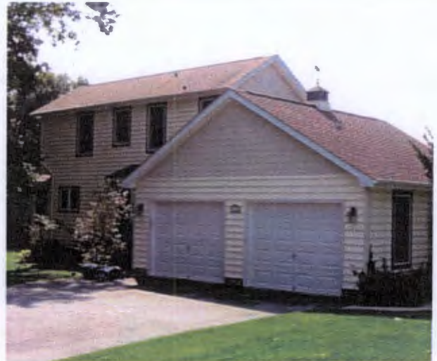
This garage addition visually dominates the historic structure.
