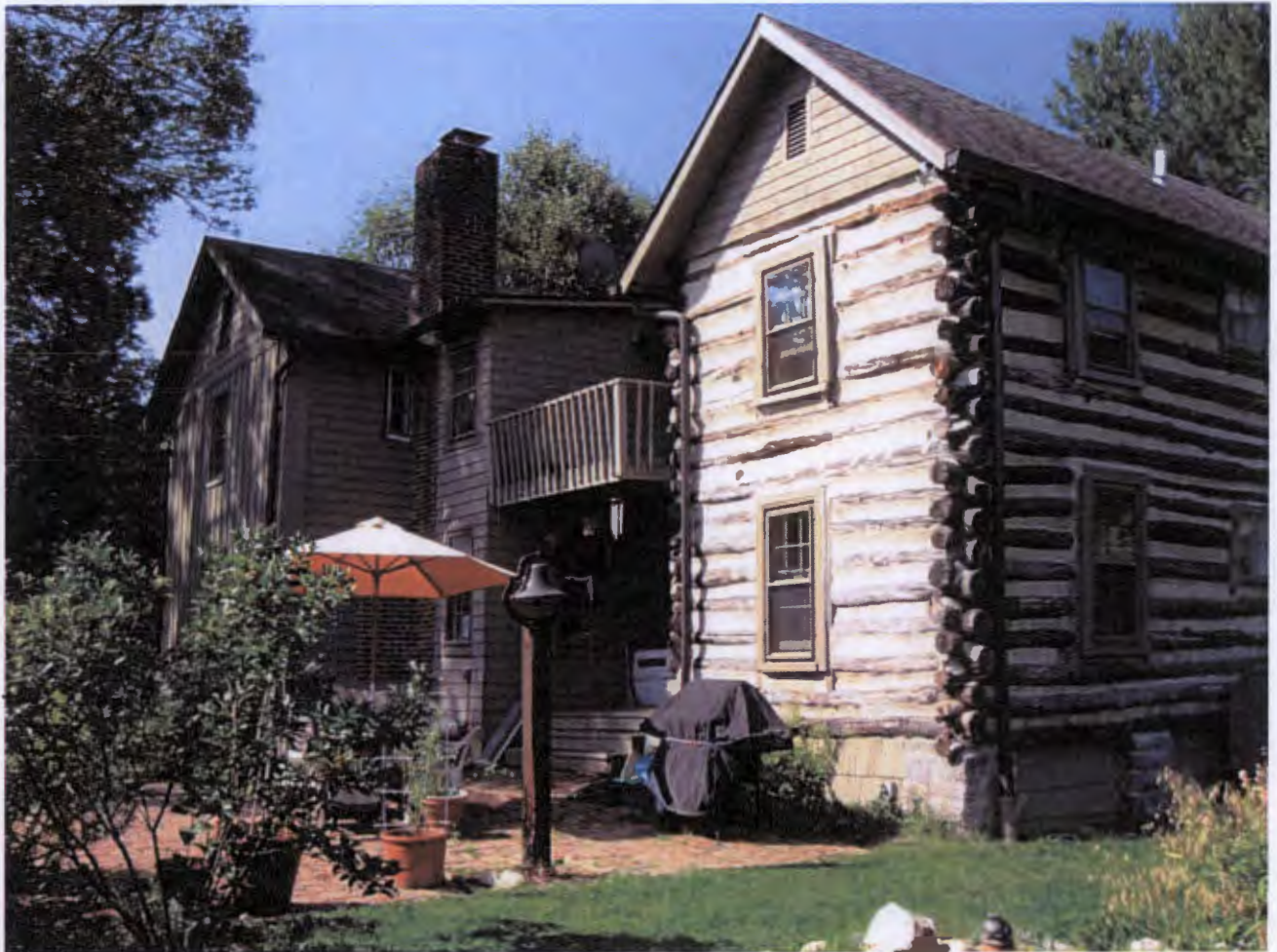
Several additions were added to this log structure, which have gained historic significance in their own right.
