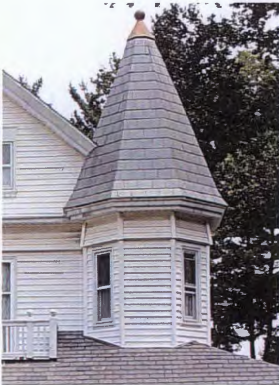
Towers are often located on top of projecting bays.
