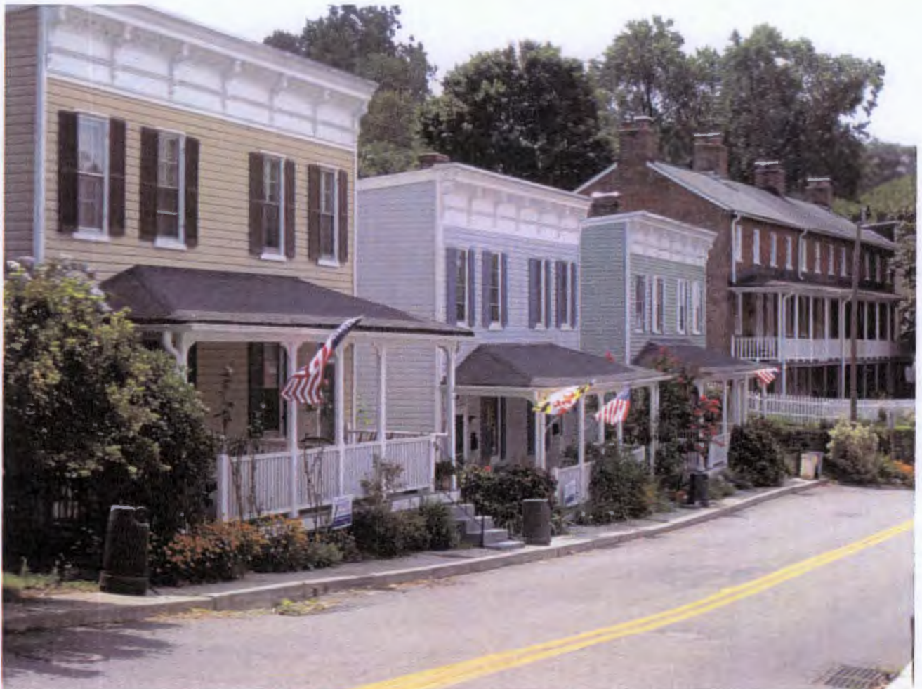
Front porches add a unifying element to the streetscape.
