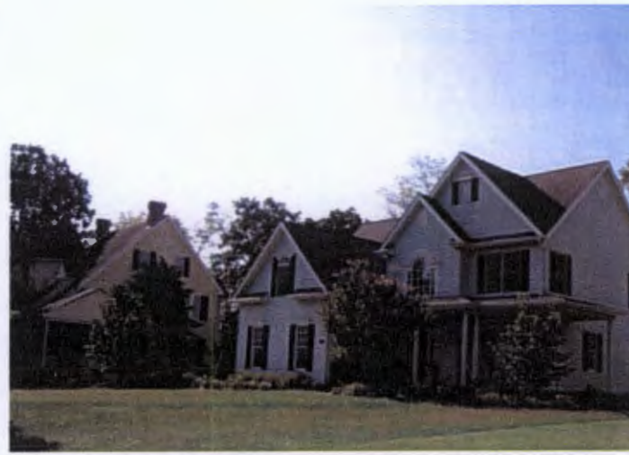
This infill structure emulates the size, scale and massing of the abutting historic structure. Prevalent design elements of the historic community are replicated in the new building and the garage is accessed from the rear.
