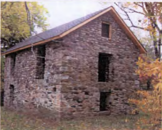
This former slave quarter was stabilized with the aid of County tax credits.
