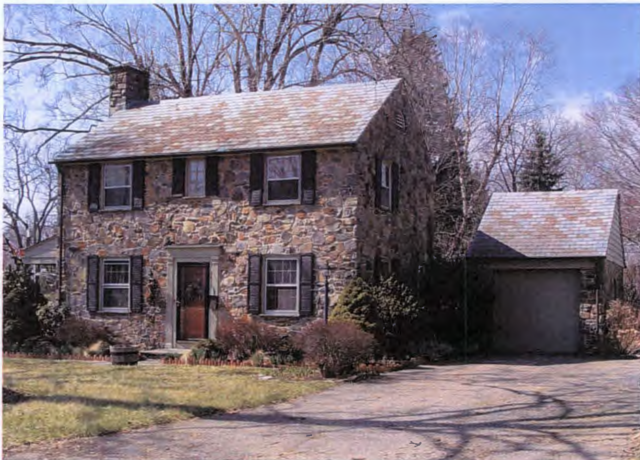
The garage shown here compliments the historic structure.
