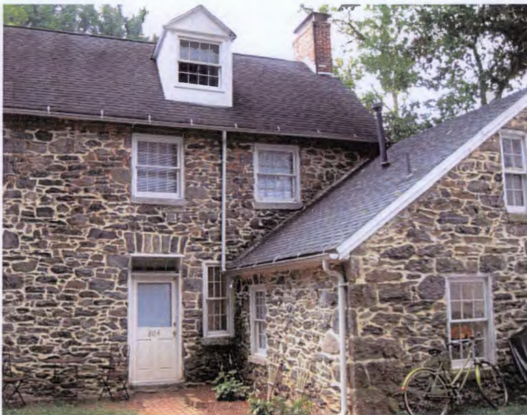
The type of stone used, how it is finished and laid, and the width, color and profile of the mortar joints all contribute to the appearance of a stonewall or above-ground foundation.
