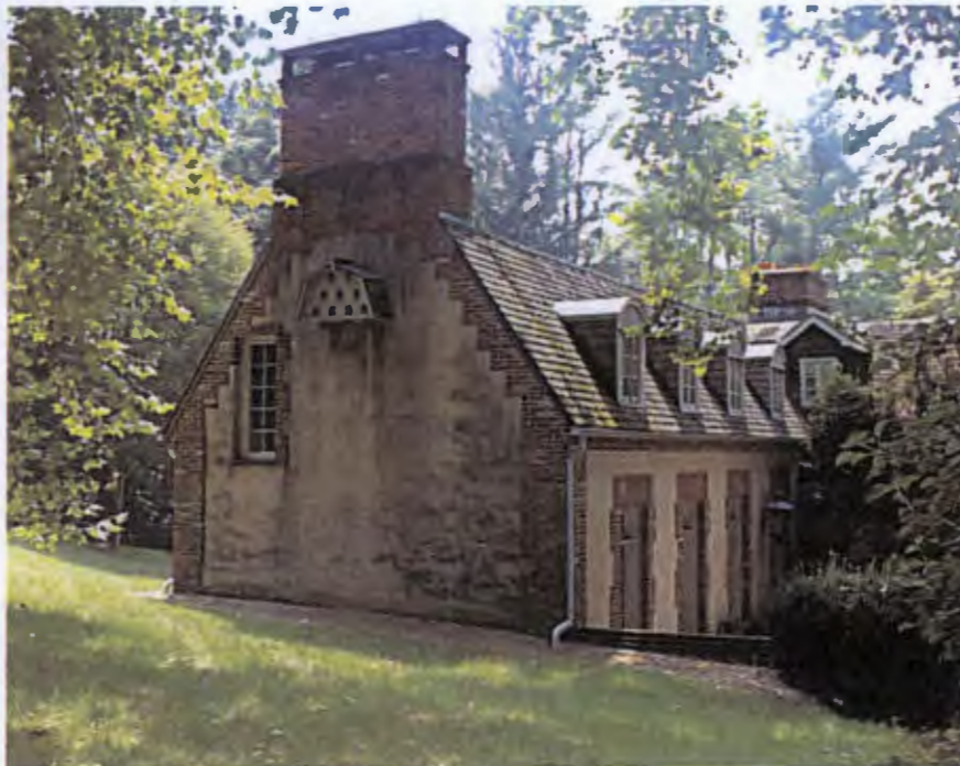
Chimneys are frequently prominent features on historic buildings.
