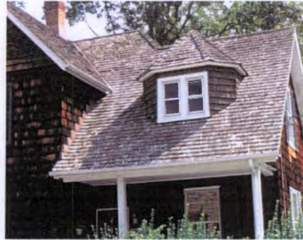
Because of fire hazards, wood shingles are no longer in frequent use.
