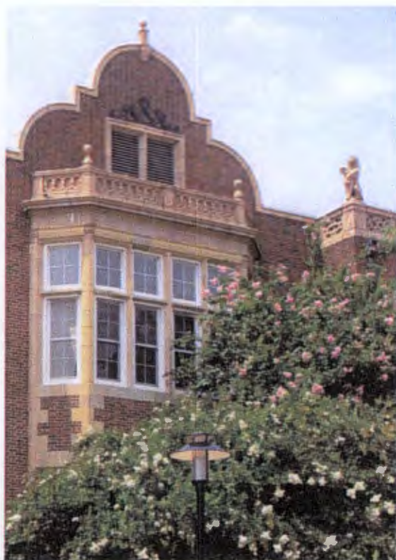
Parapets are generally designed to give a building greater visual height.
