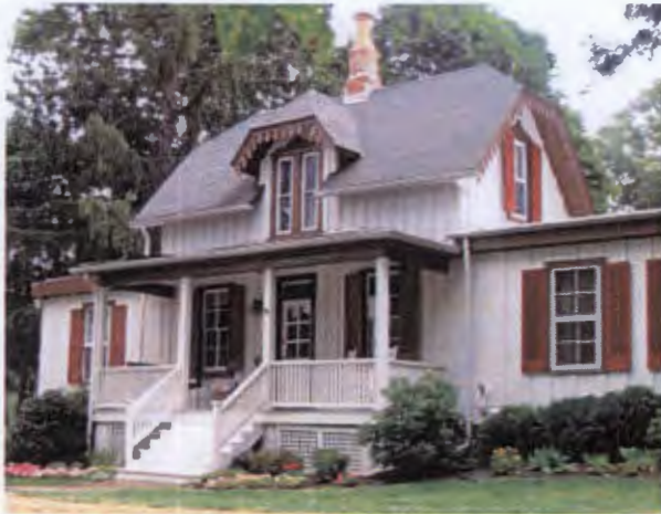
Vertical siding such as the board and batten siding is rare.
