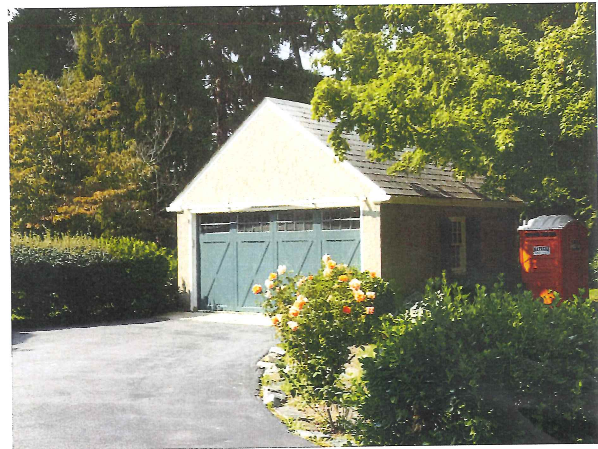
VIEW OF EXISTING GARAGE
