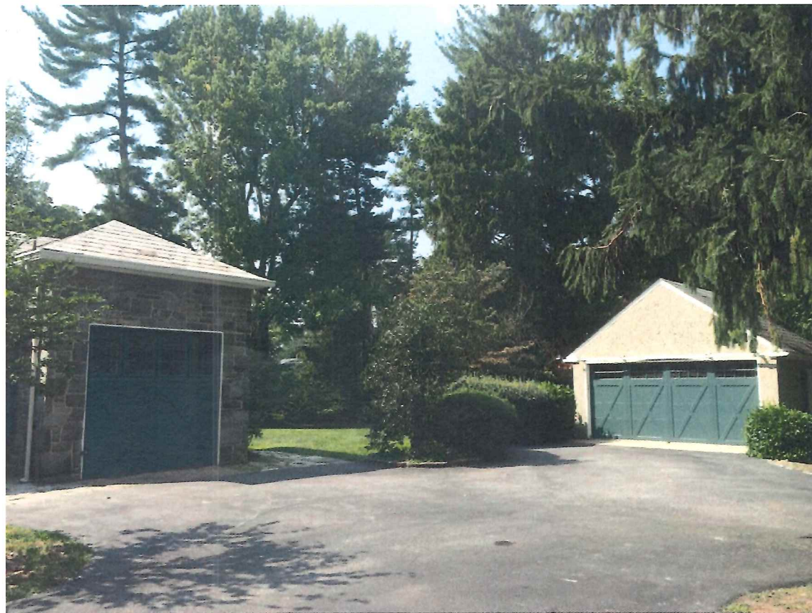
VIEW FROM SOUTHEAST CORNER OF PROPERTY
