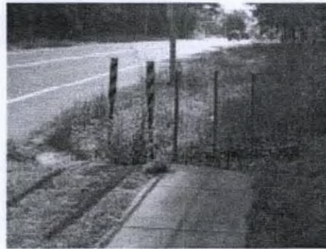
A sidewalk gap on Ebenezer Road
