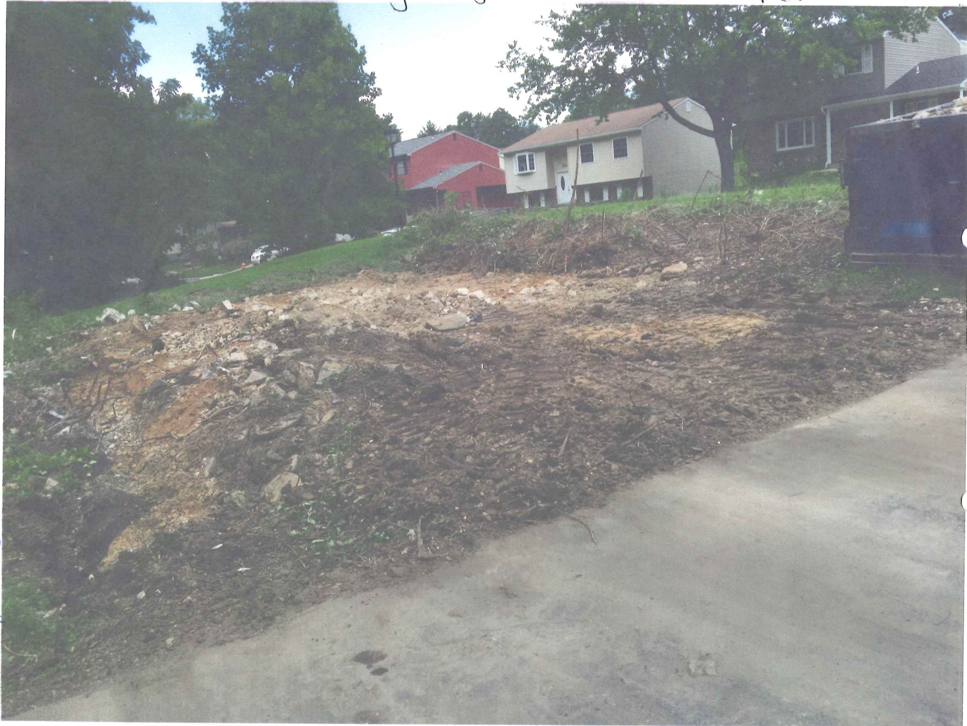
Removal of building that fell down. Neighbors across the street
