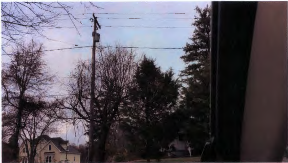
Picture 14 – 3 phase to the east of Bradshaw Road
