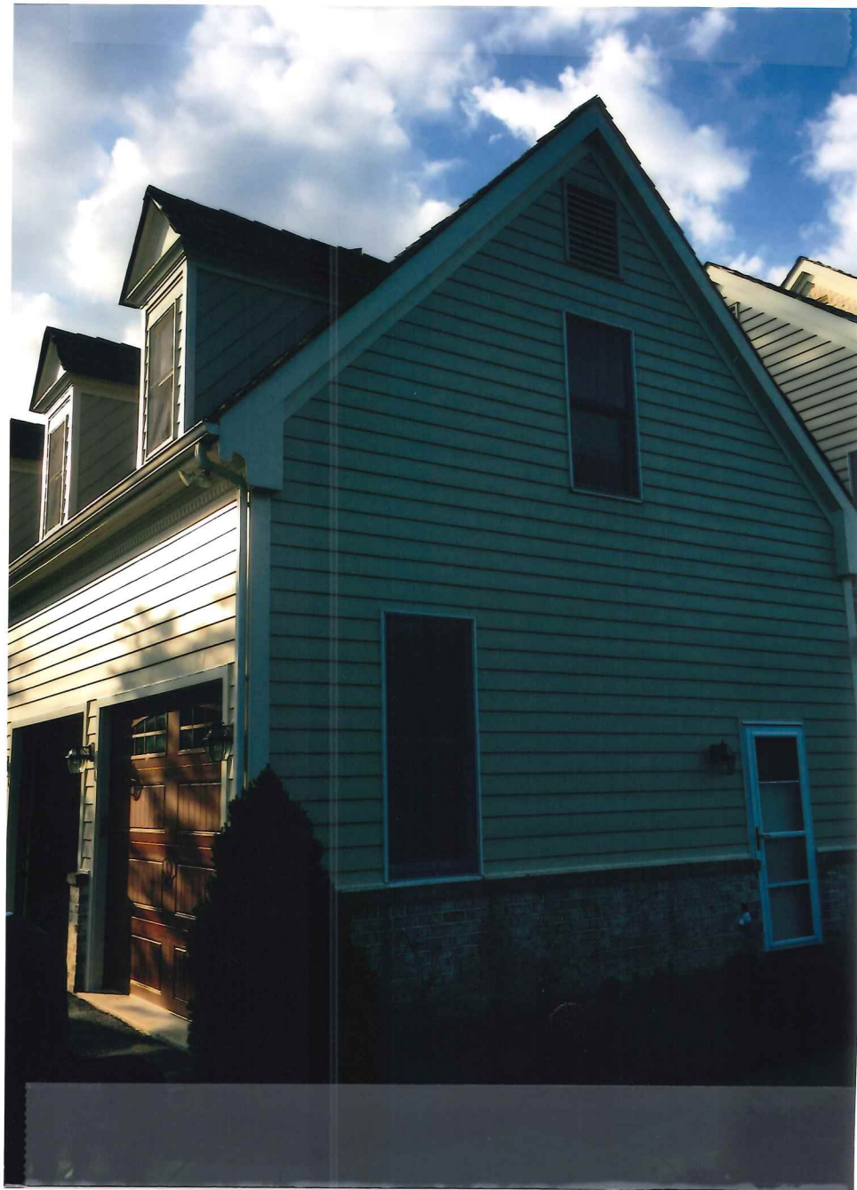
Close up of side of Garage
