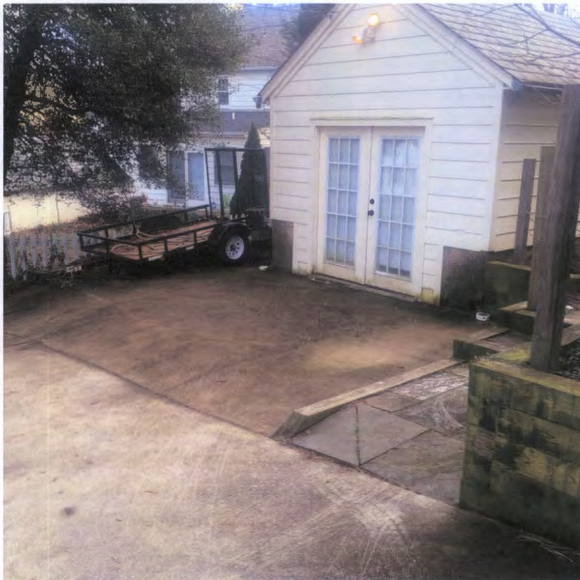
Garage connected to house and converted to living space.
