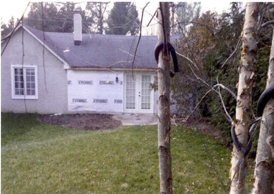
View west towards proposed Covered Porch from 1512 Maywood Avenue
