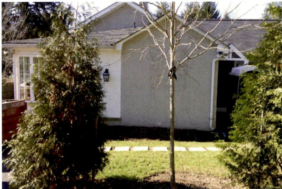
View west towards proposed Carport from 1512 Maywood Avenue
