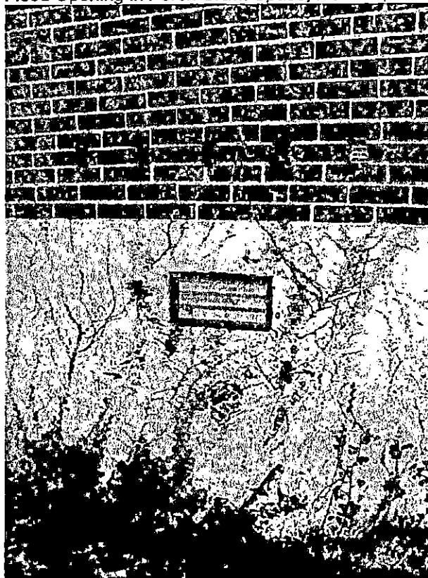
Flood Opening in Porch Crawl Space, March 4, 2016
