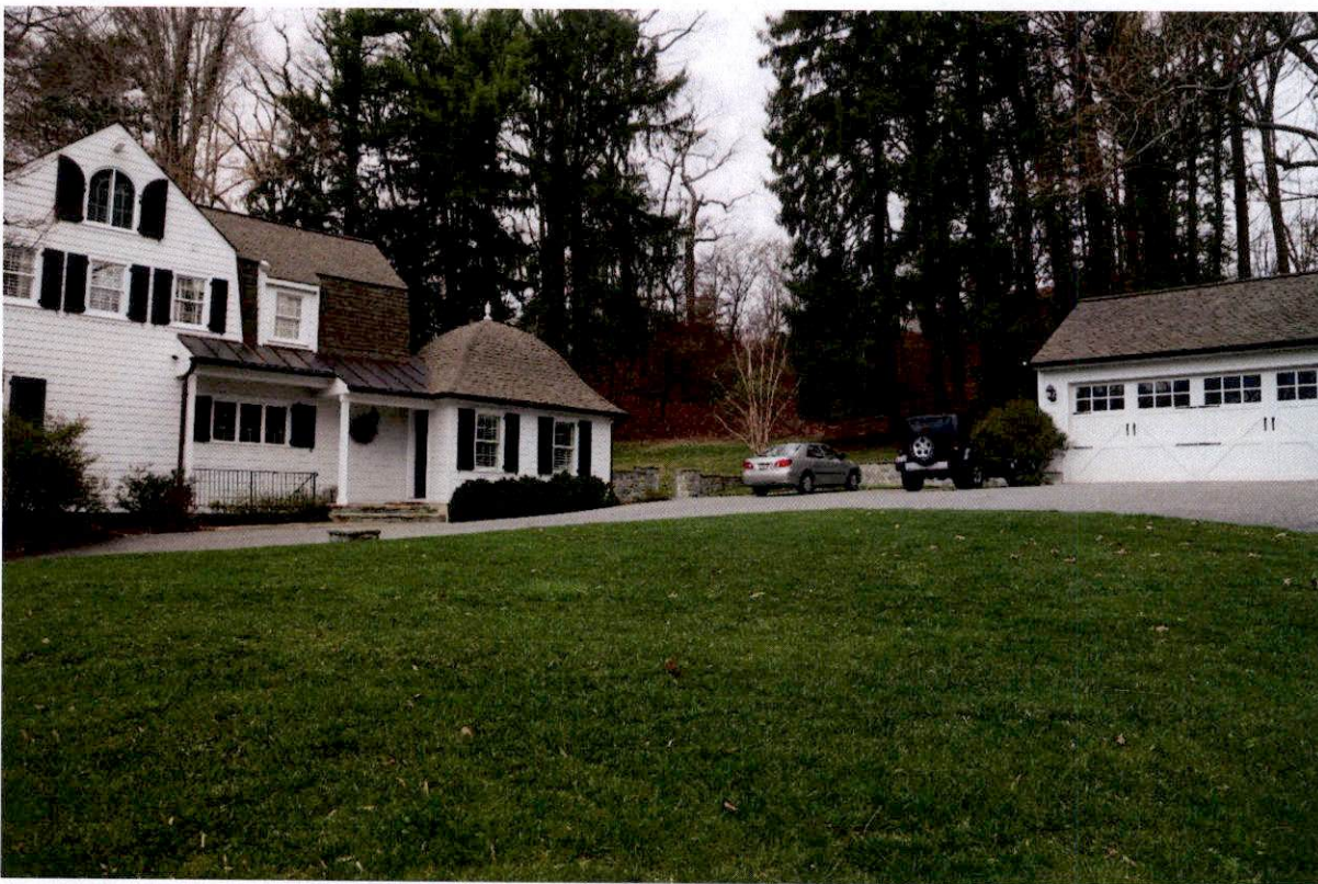
Photograph #6 - View from driveway island with site for Accessory Bldg "A" at center behind car
