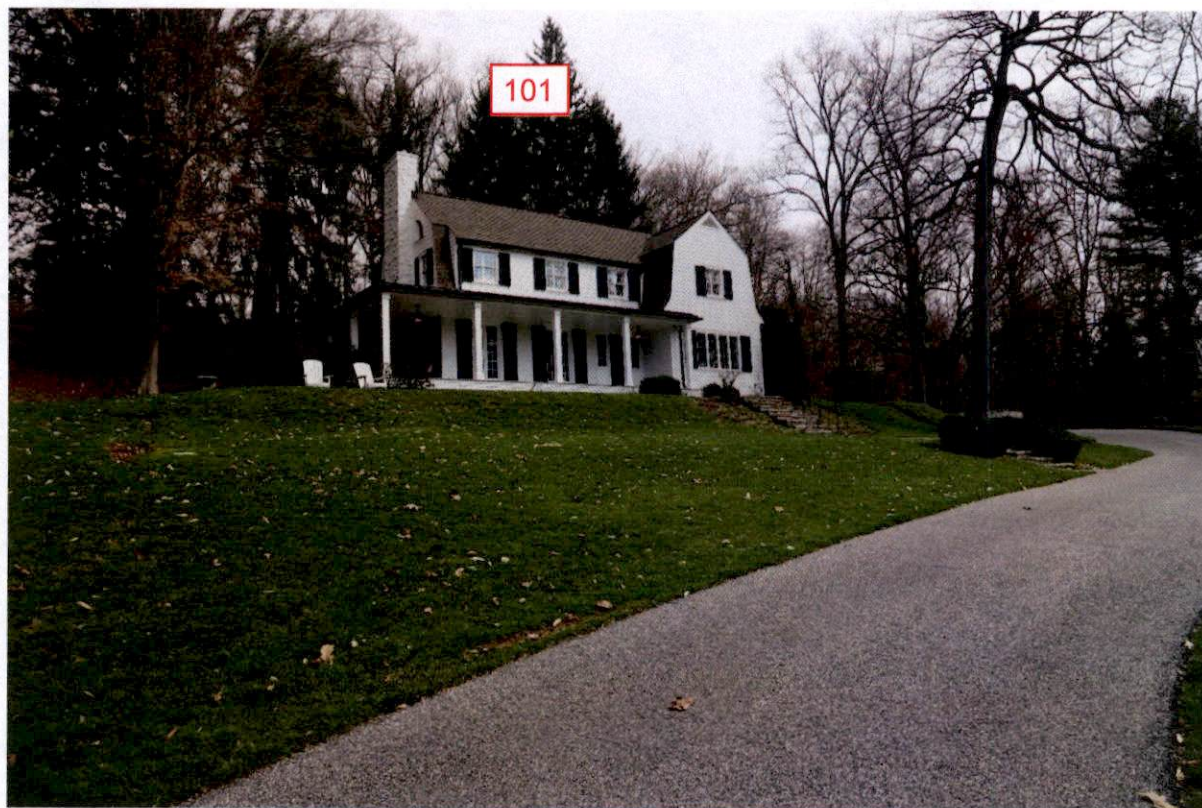
Photograph #3 - View from driveway with front and west side visible.
