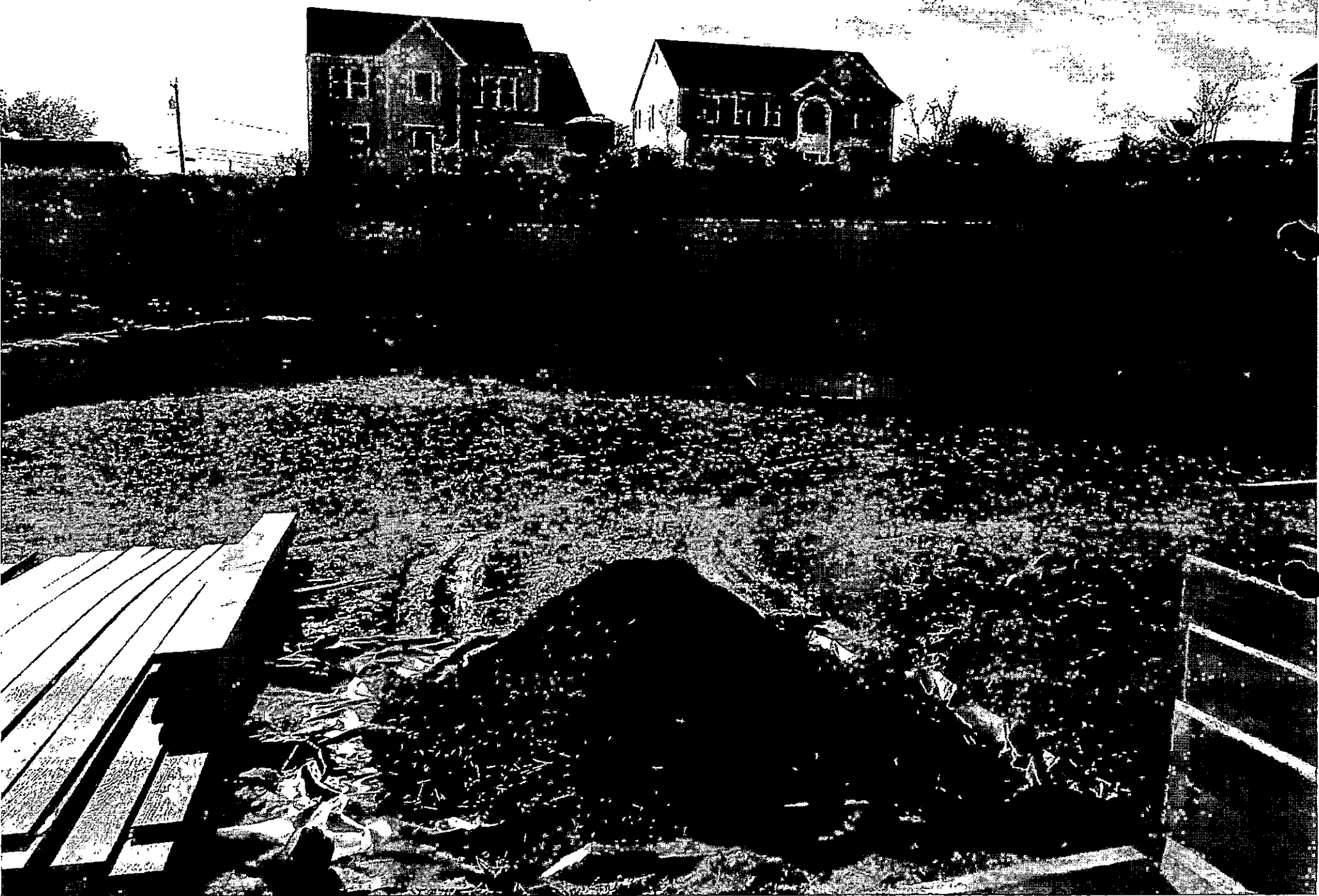
Photo 4:- Open Back Area.
