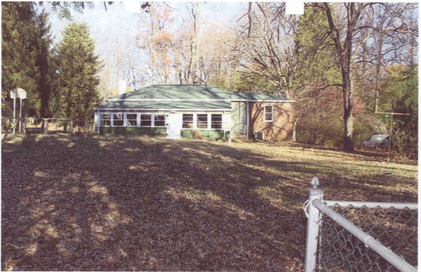
Subject property from the South
