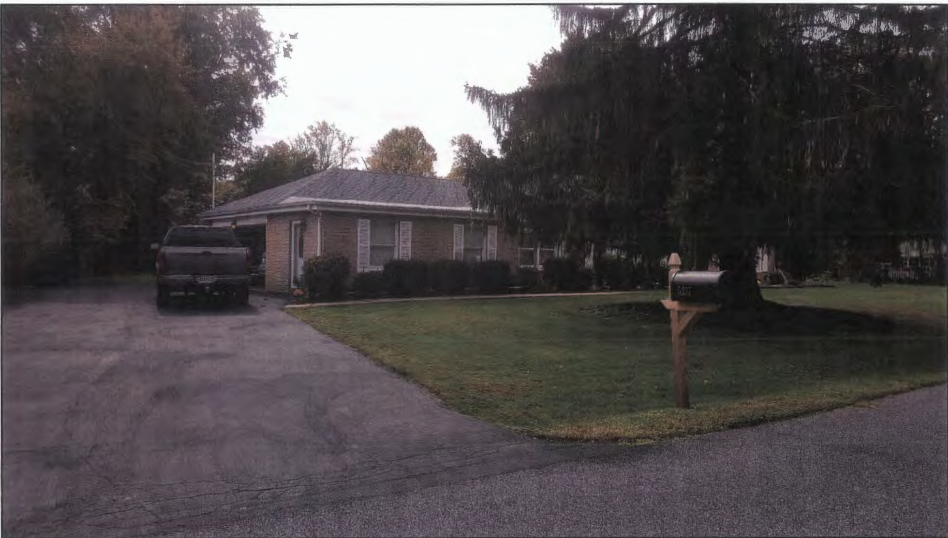
①⑧ #5217 BANGERT STREET
