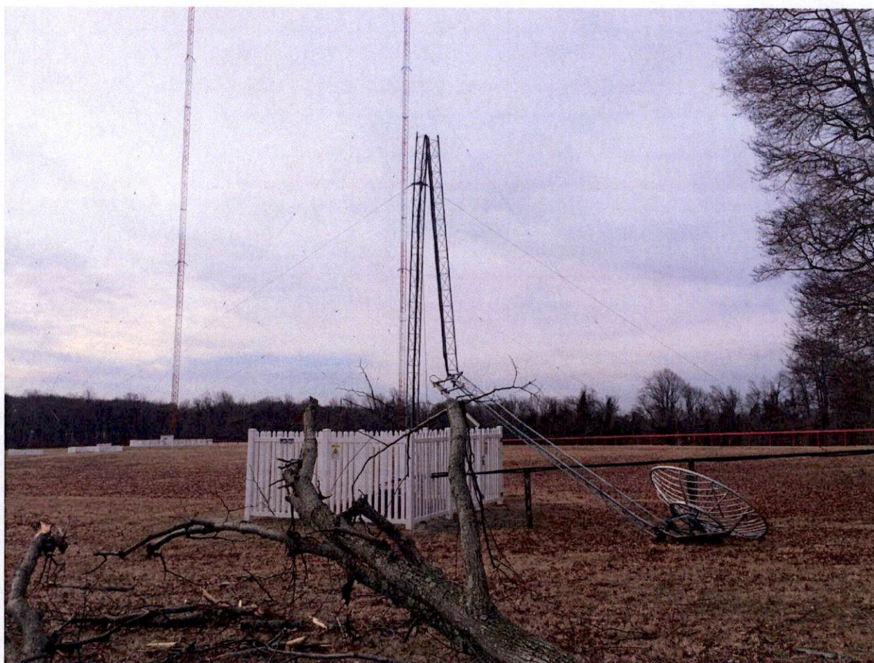
Photo 4 of 4 (damaged in storm April 2015)
