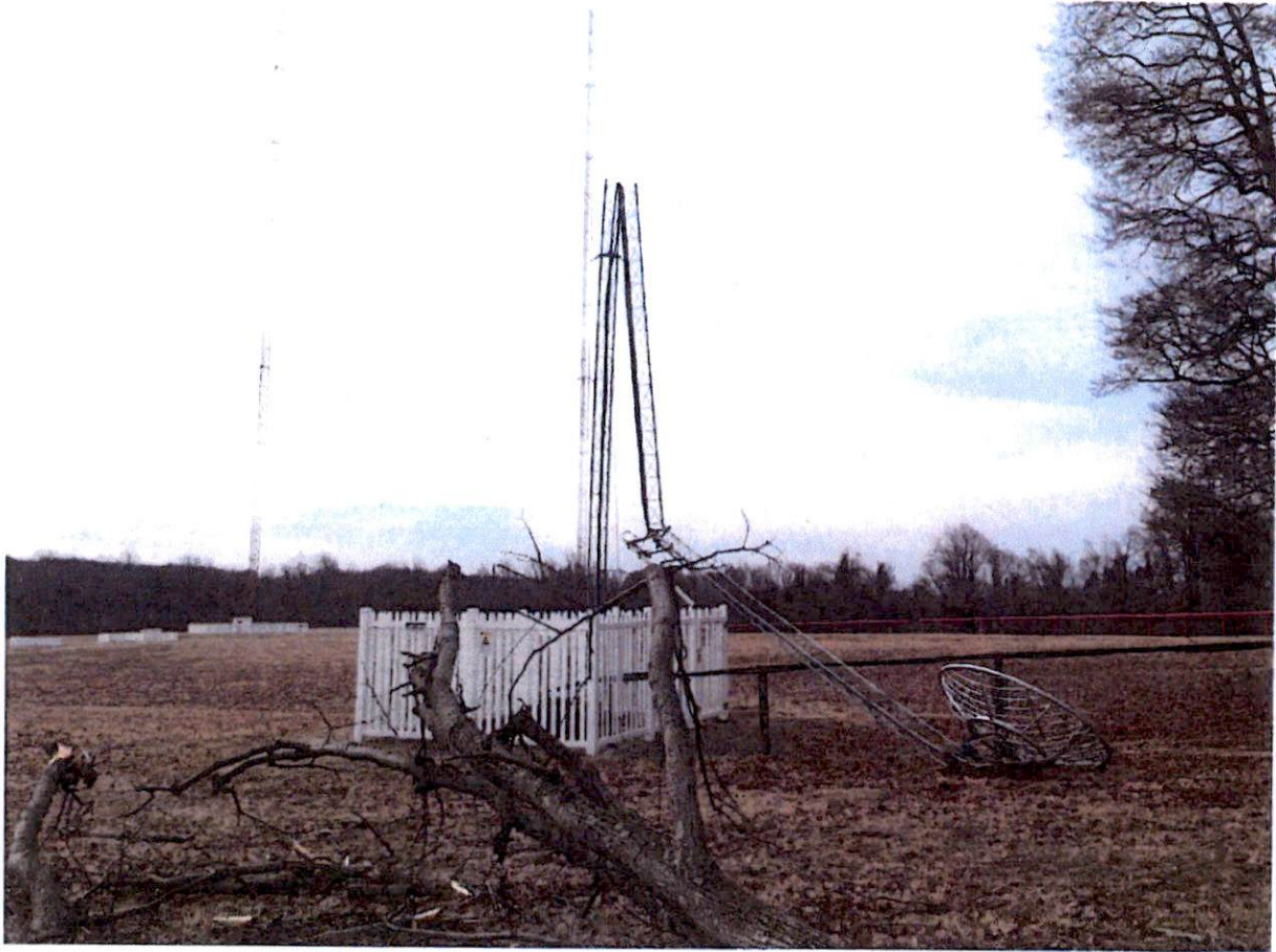
Photo 4 of 4 (damaged in storm April 2015)
