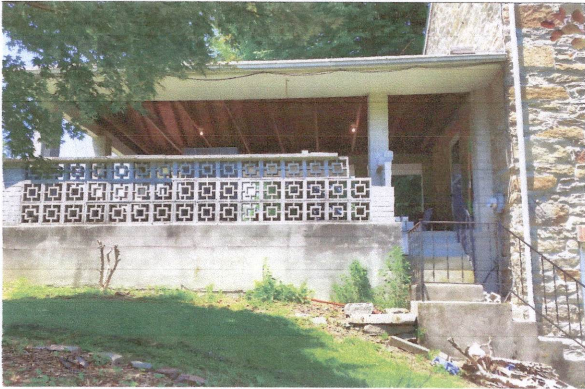
11909 WOODBERRY PLACE CARPORT: BACK (LOOKING NORTH)
