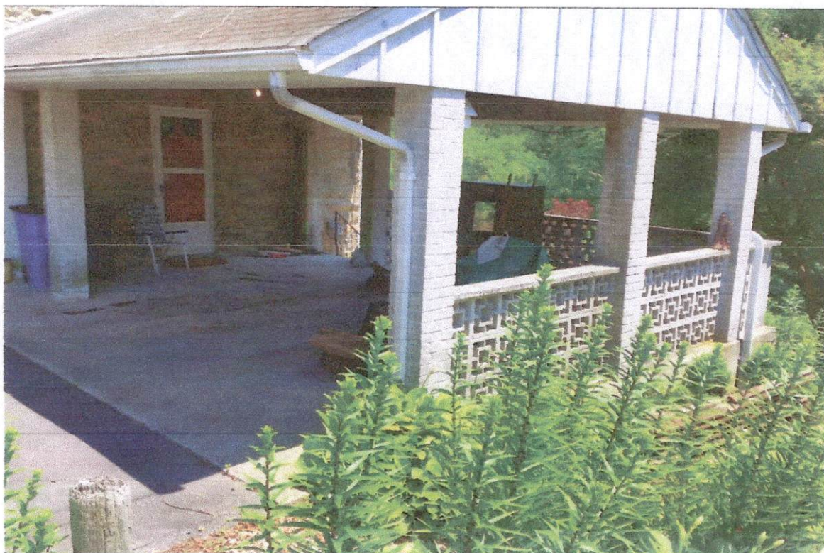
11909 WOODBERRY PLACE CARPORT: SIDE #1
