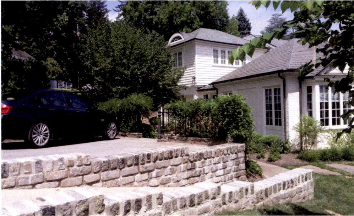
G – View north from side of proposed Garage towards the property Owner's house
