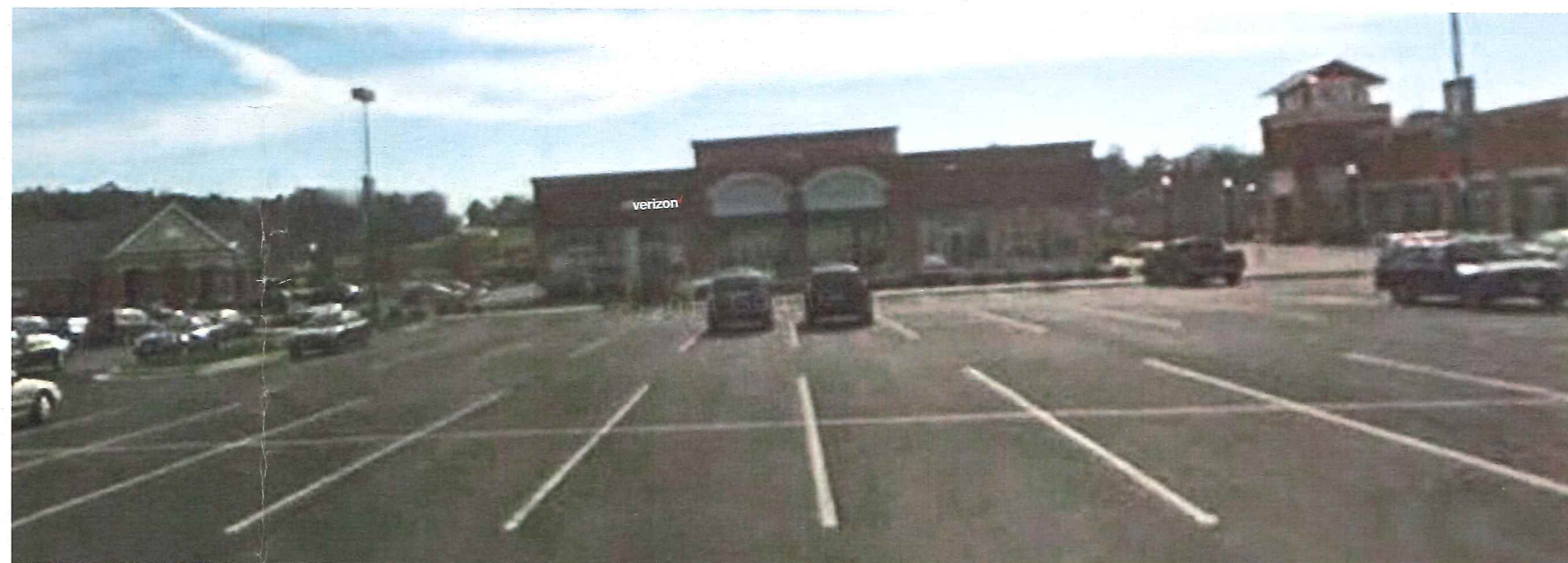
Back of Store from Parking Lot (directly behind store)
