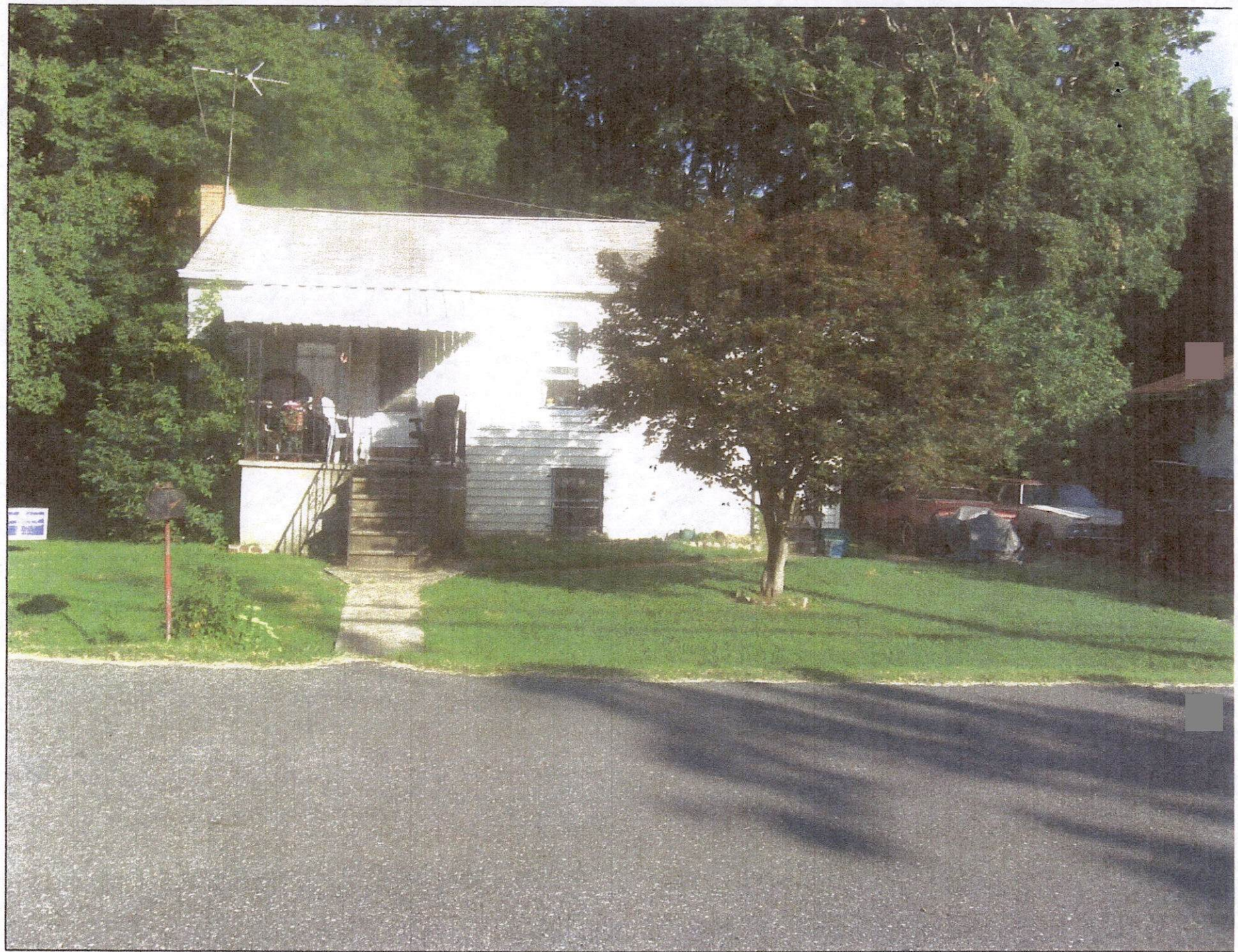
①9 #8214 ROSEBANK AVENUE—RESIDENTIAL
