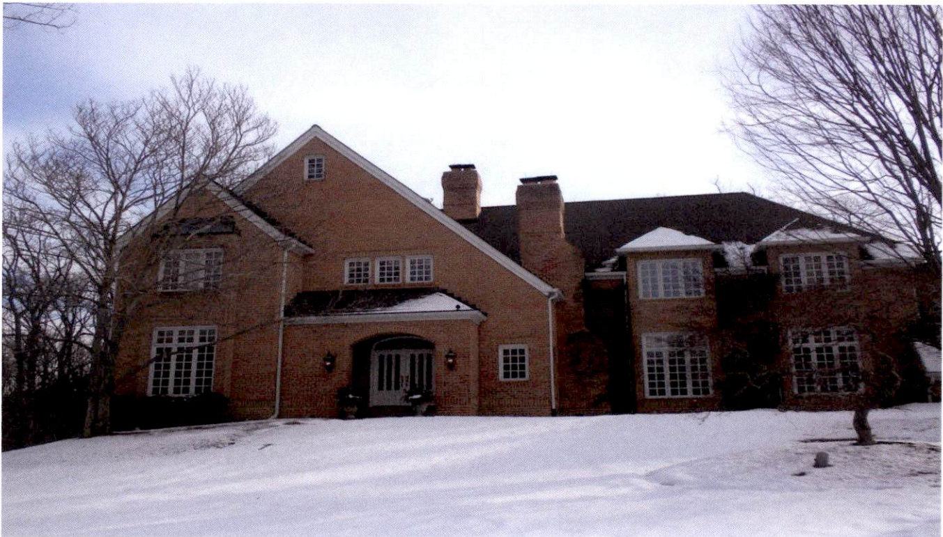
2/ Detail view of existing house to illustrate roof lines and height of structure
