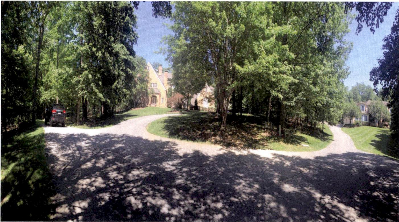
1/ View east from Cleghorn Road towards existing house, proposed garage on the right rear, and pool house and pergola/storage structure to the left rear
