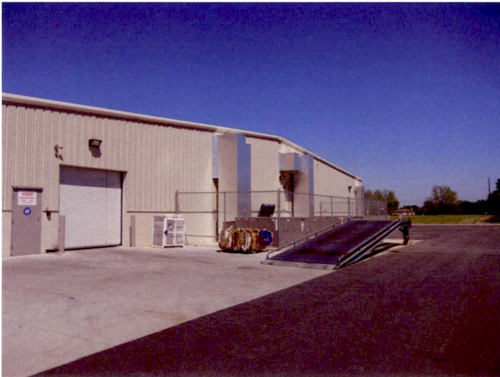
Loading Dock and Ramp
