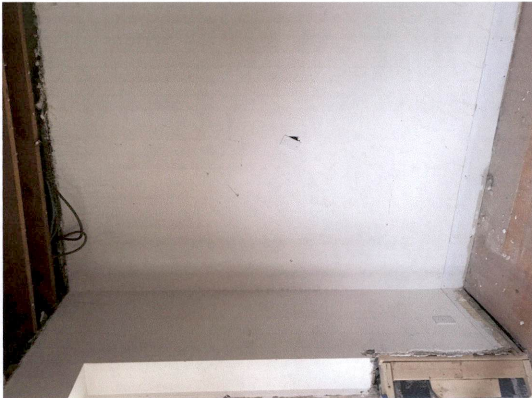
Back side of front door hall/ stair in first floor apartment
