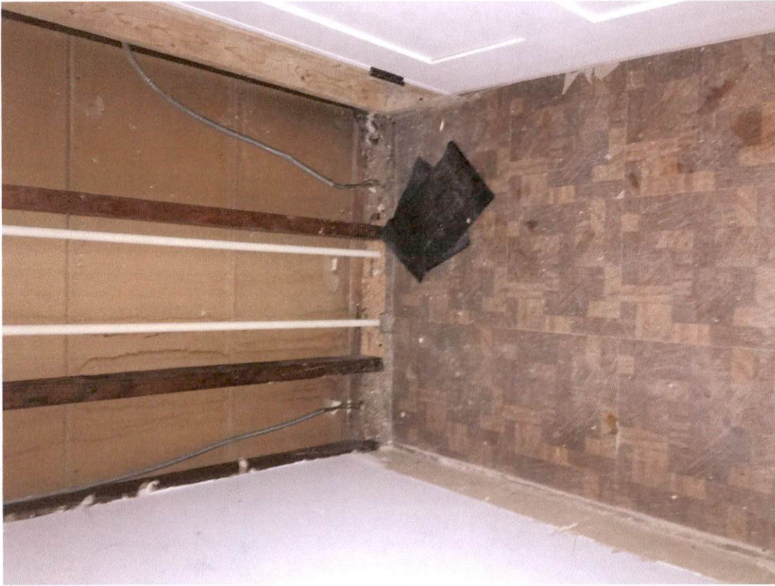
Inside first floor front door hall/ stair to second floor
