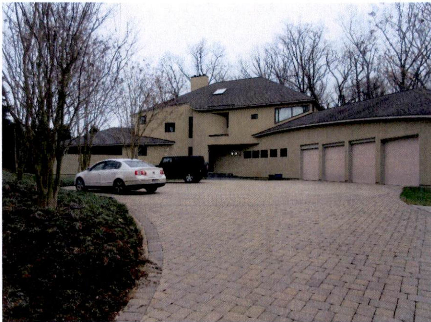
Looking east from driveway entrance off road towards existing house.
