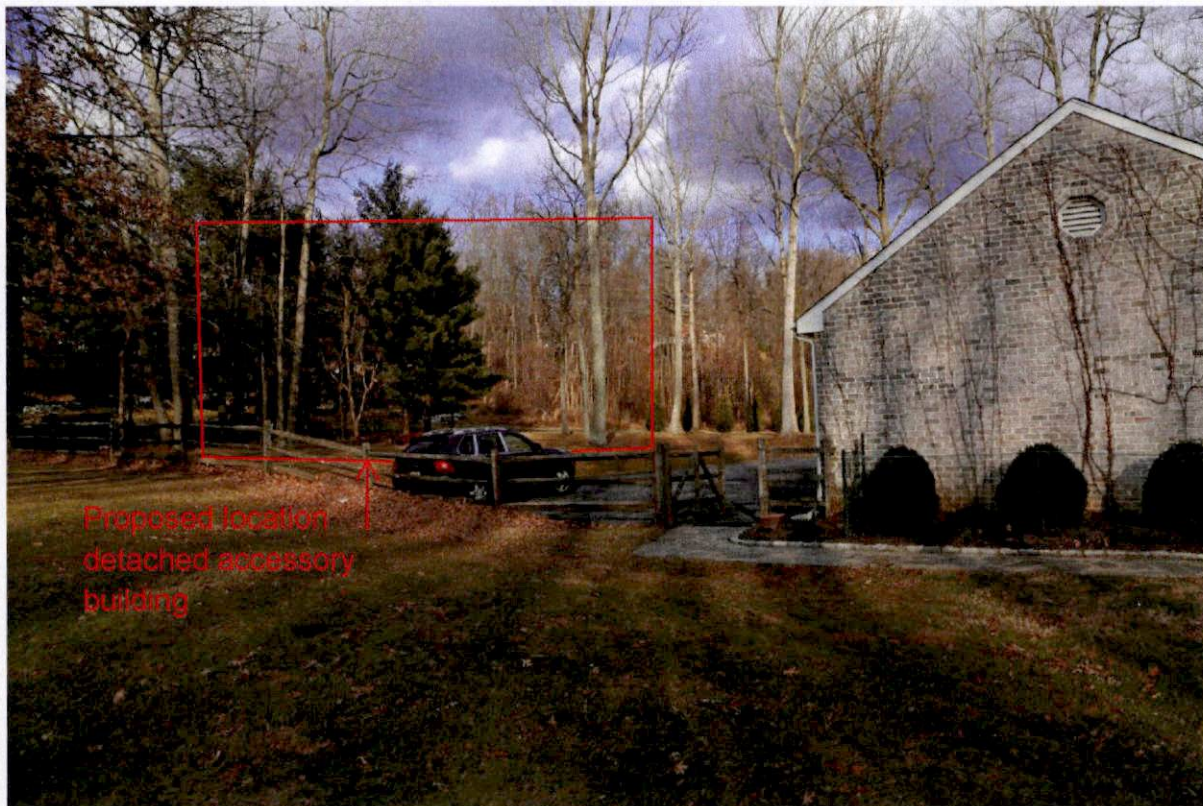
Photograph #6 - View looking north from rear yard
