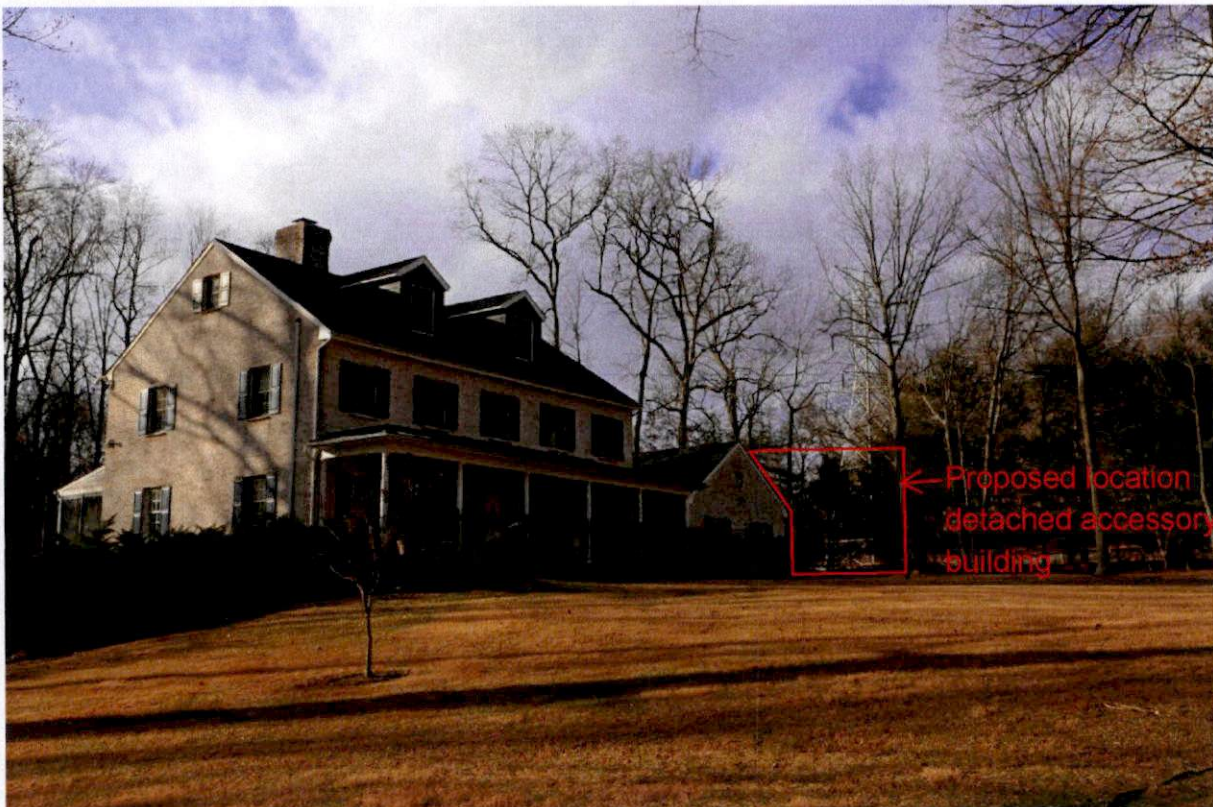
Photograph #2- View from southeast from front yard
