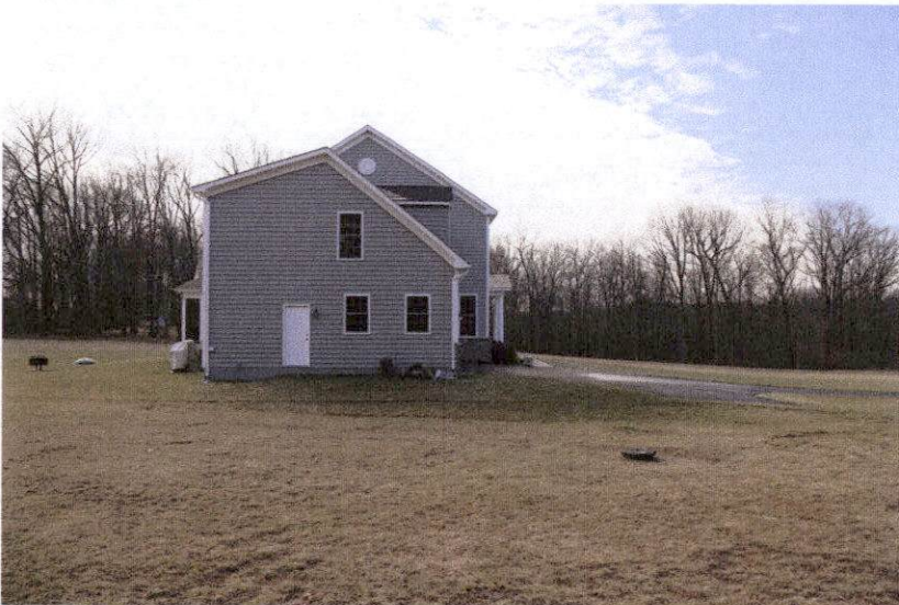
left side of house, you can see the black cap of the Propane tank in the ground.
