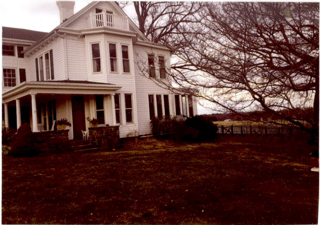
South (front) of existing residence.
