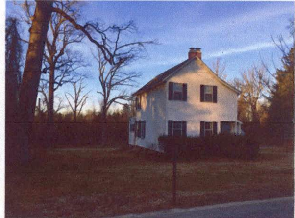
Current view of property from Windsor Rd
