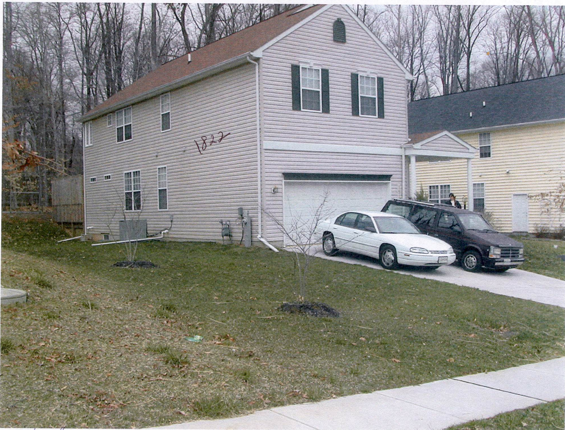
Item #0239 Reflects location of addition on left side of picture - 1822 Cainewood Ct.
