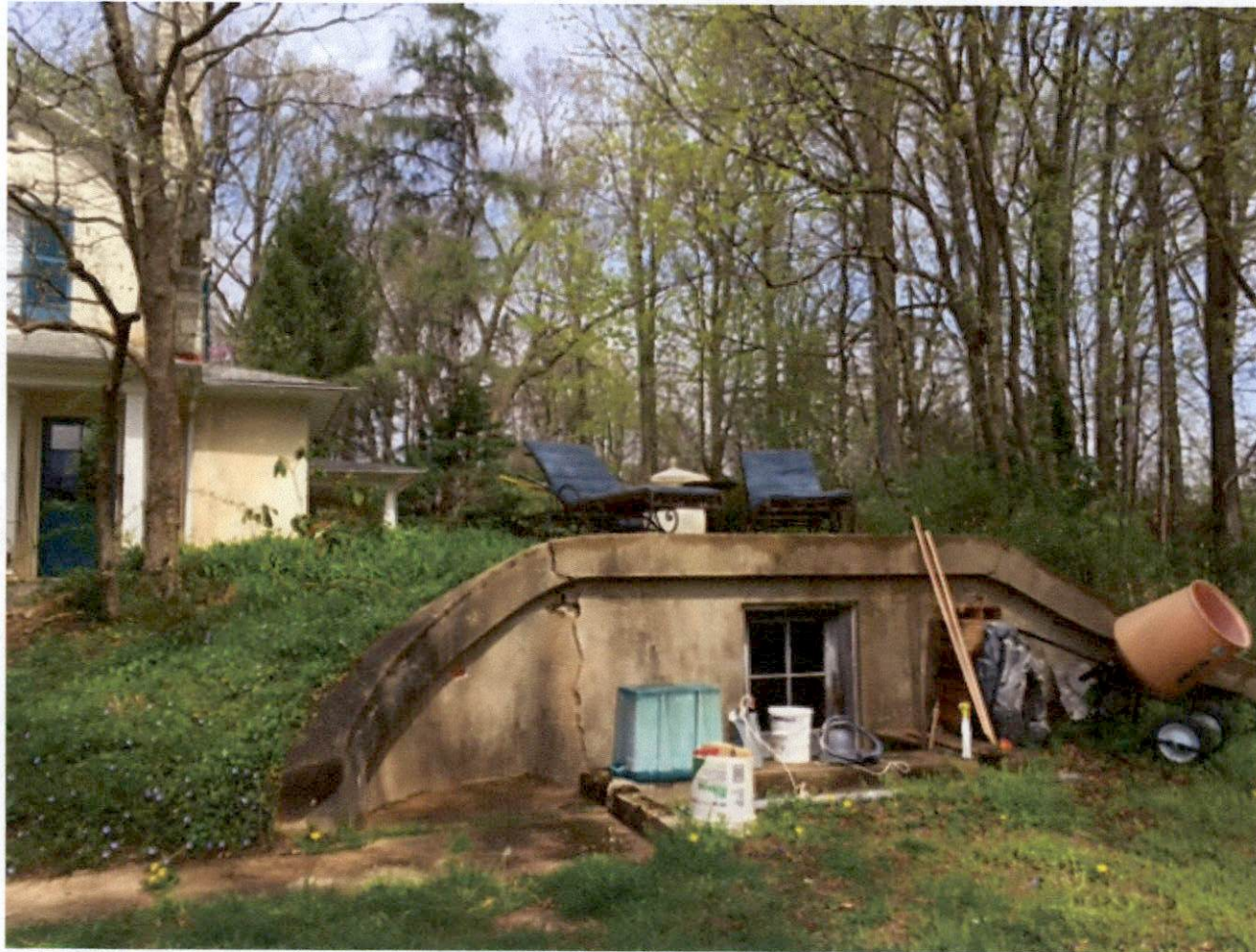
Well house located on side / back of house
