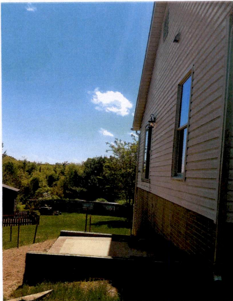
CLOSE VIEW OF SIDE (EASTSIDE) OF PROPERTY. LOOKING SOUTH FROM FRONT YARD.
