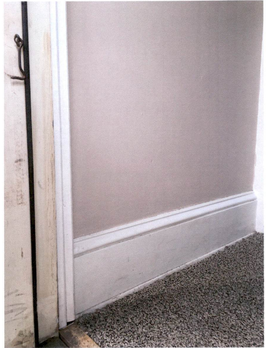
ENTRANCE TO SECOND FLOOR APARTMENT AT TOP OF STAIRS (AS SHOWN LEFT)
