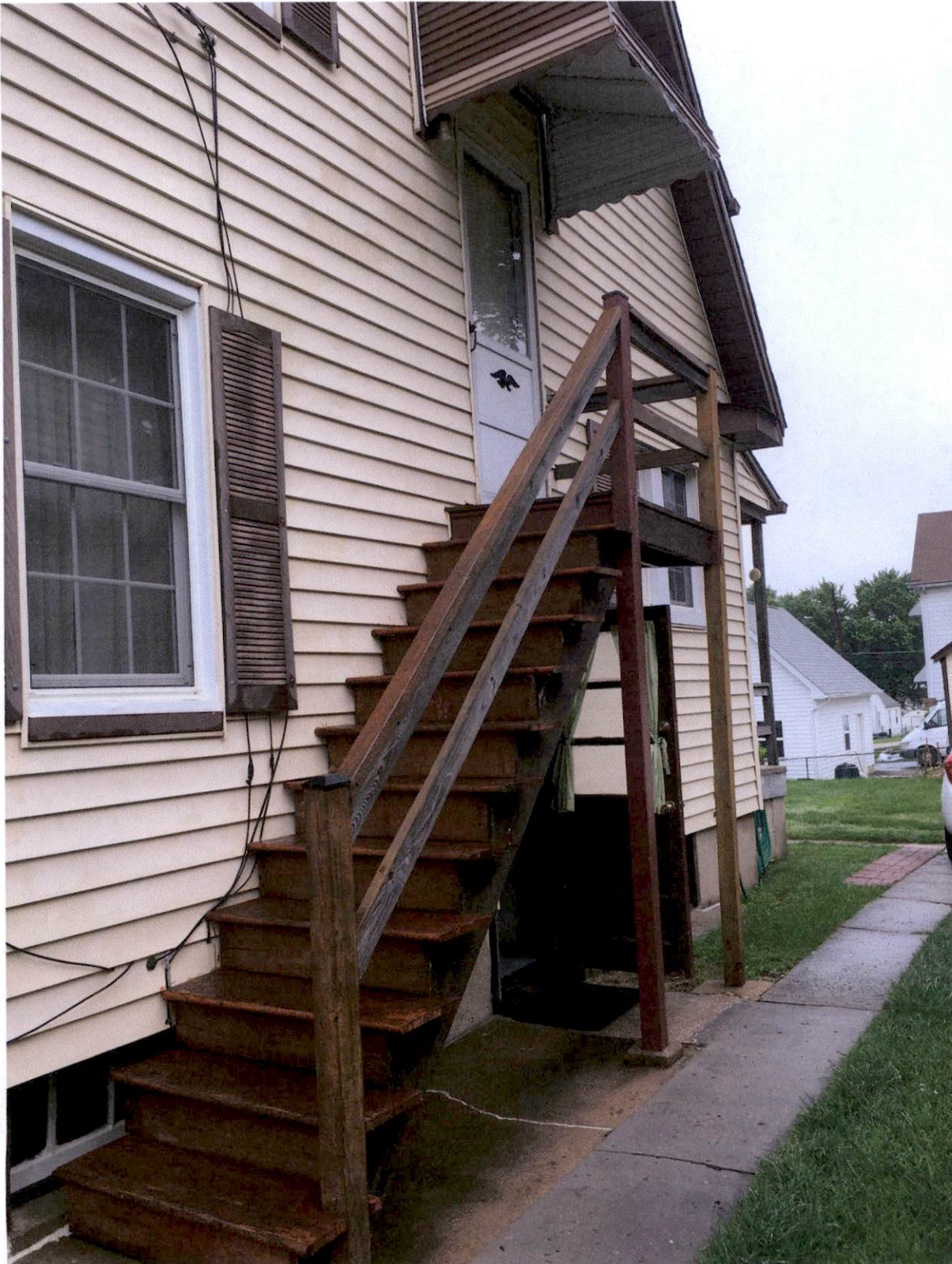
Entrance to second floor apartment 4502 Ridge Avenue
