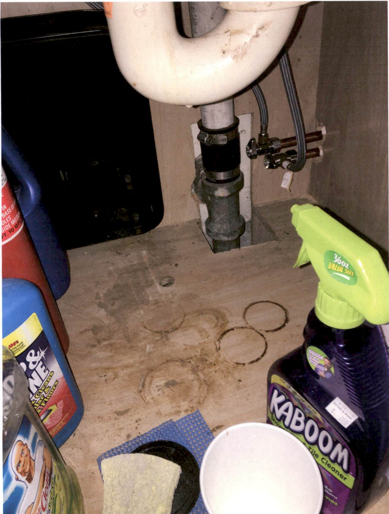
Under kitchen sink on upstairs apartment. Cast steel waste pipe
