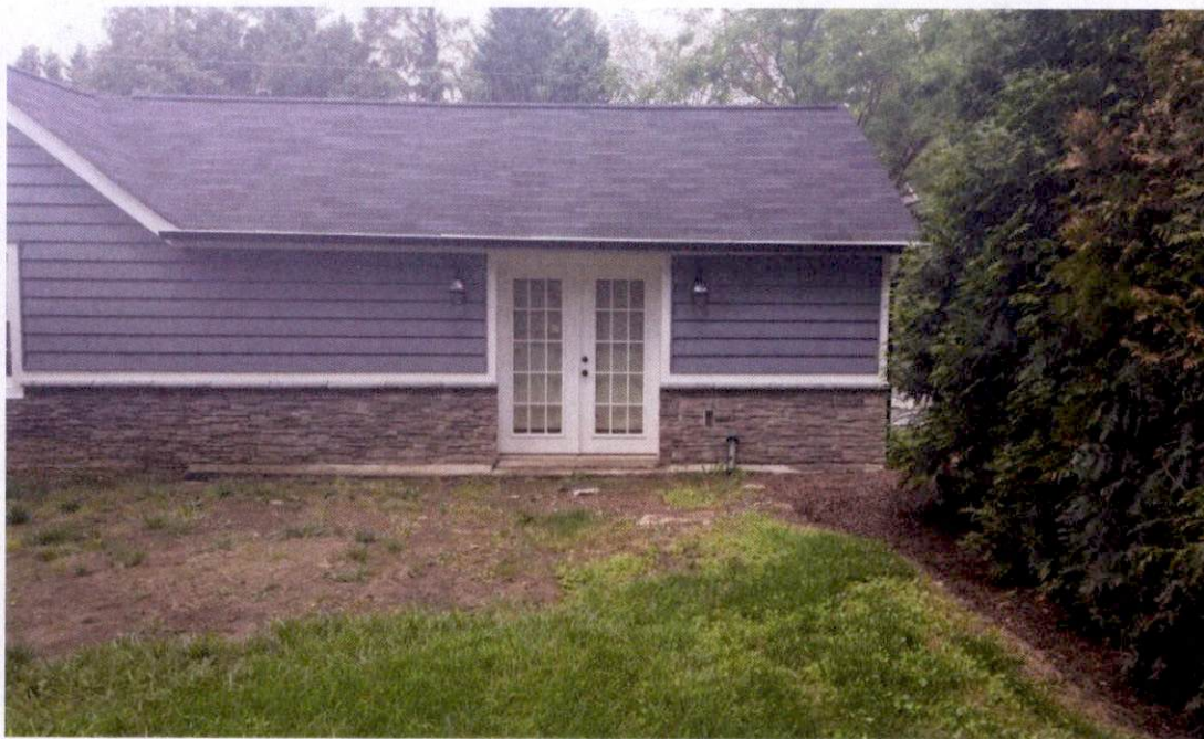
6 - View west from proposed Garage towards House
