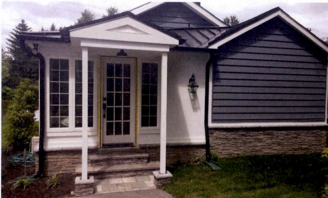
2 - View west towards the relocated front door of the House
