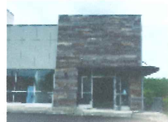
EXISTING STORE FRONT
