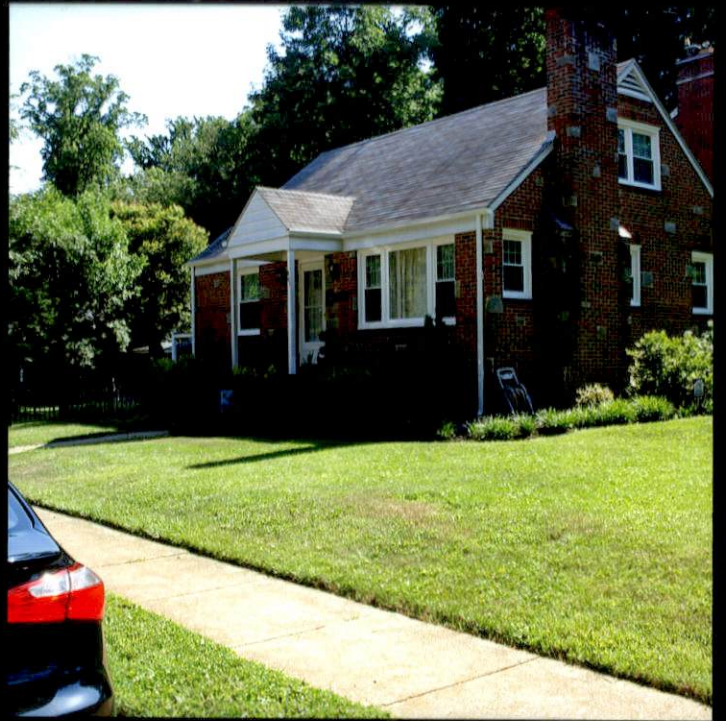
601 UPLAND ROAD, CORNER OF UPLAND ROAD AND GLENROCK ROAD
