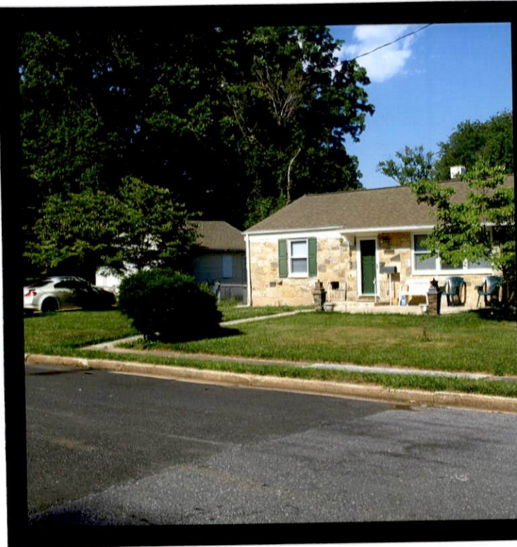
716 MILFORD MILL ROAD, CORNER OF CYLBURN + MILFORD MILL ROAD
