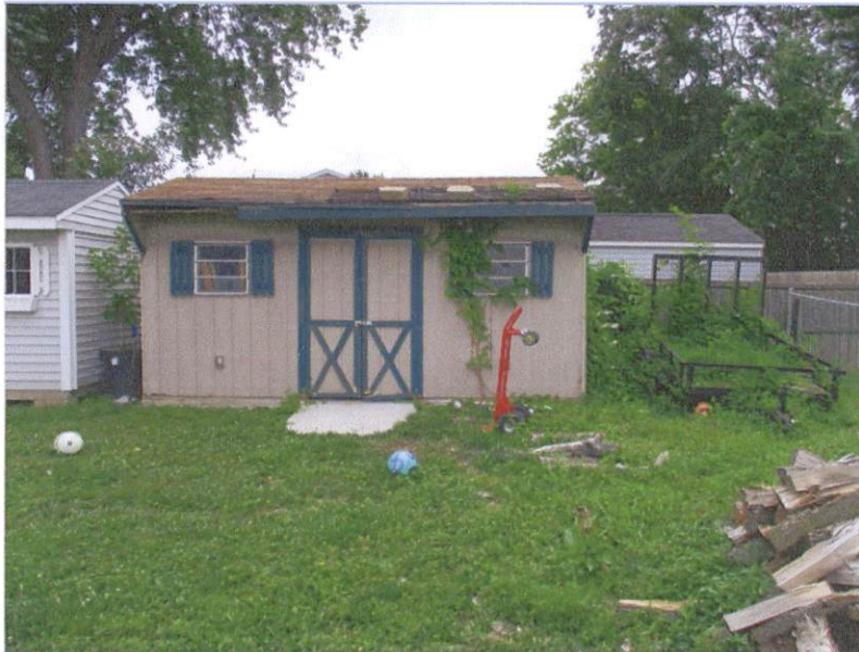
EXISTING SHED TO BE RAZED
