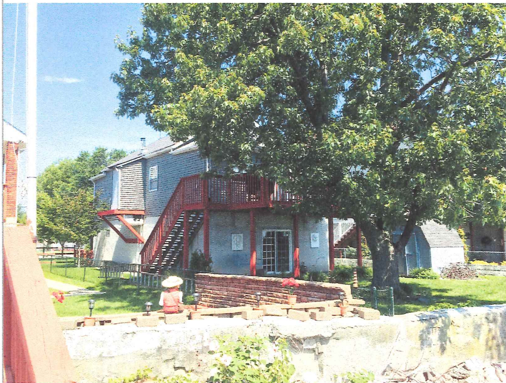
7212 RIVER DRIVE RD. REAR ELEVATION
