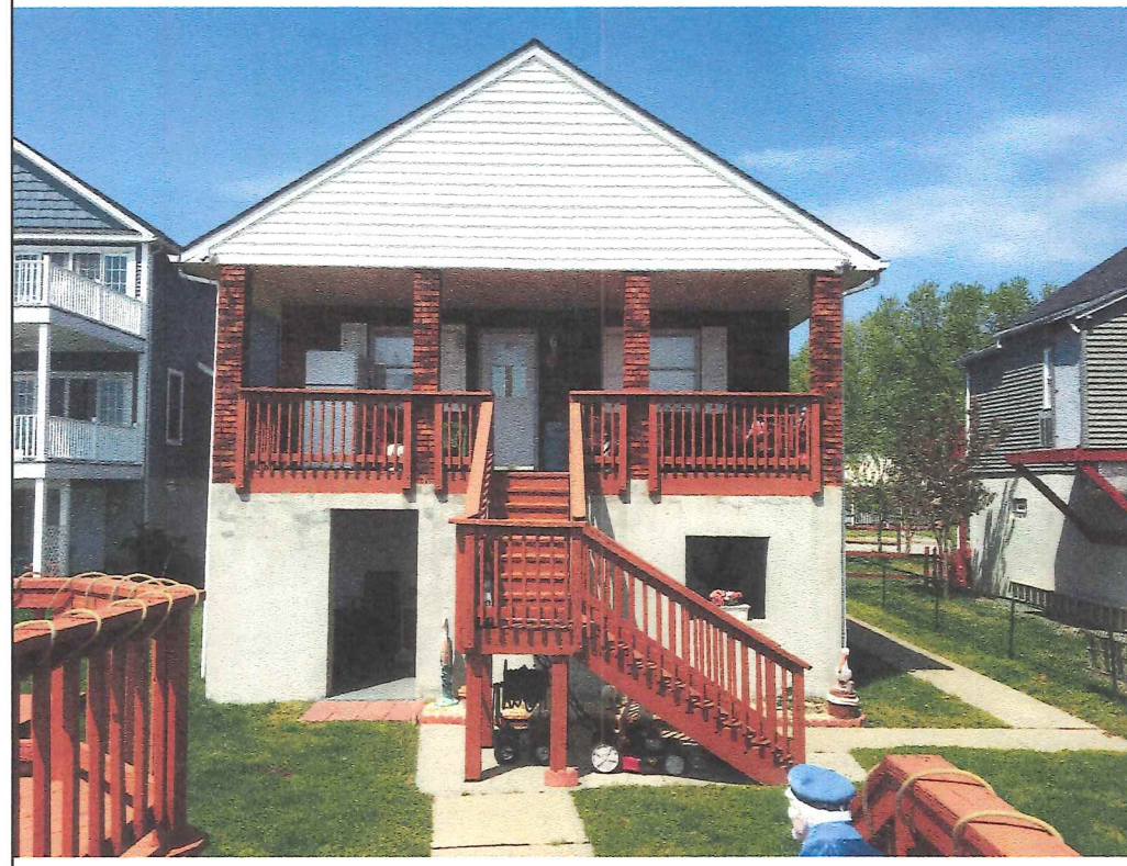
7214 RIVER DRIVE RD. REAR ELEVATION
