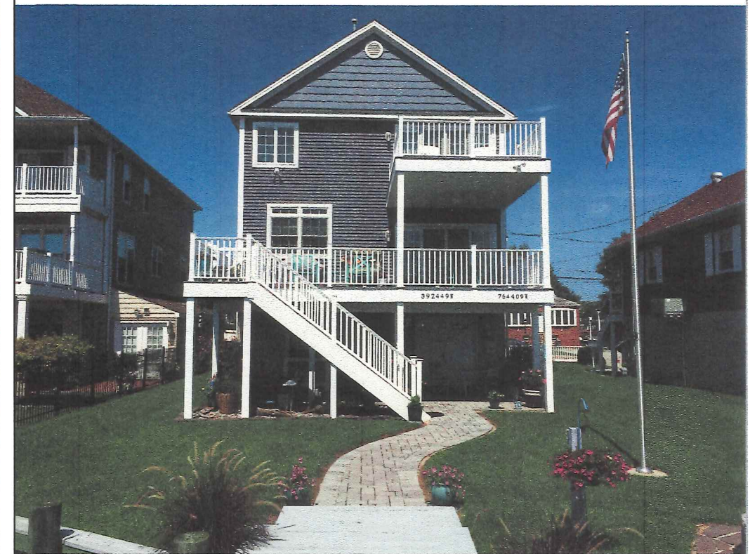
7216 RIVER DRIVE RD. REAR ELEVATION
