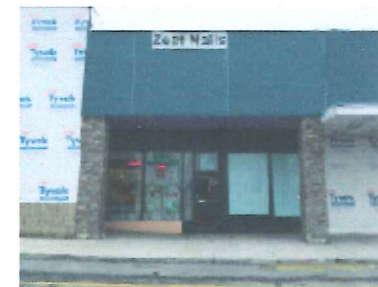
EXISTING STORE FRONT
