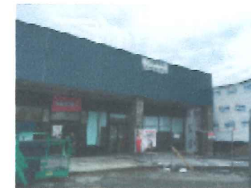
EXISTING STORE FRONT
