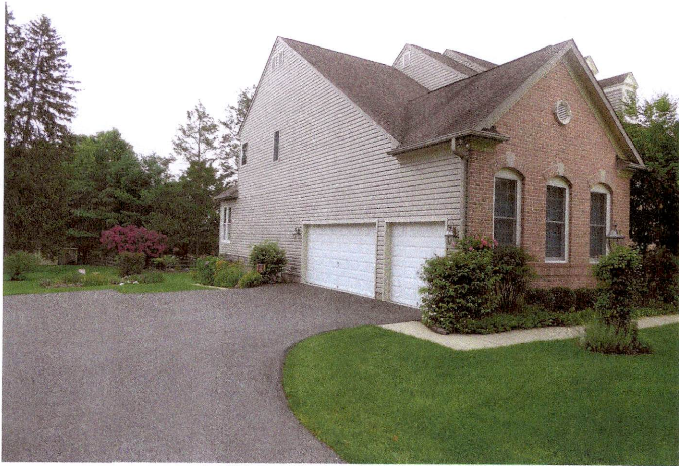
NORTH AND WEST SIDE OF HOUSE
