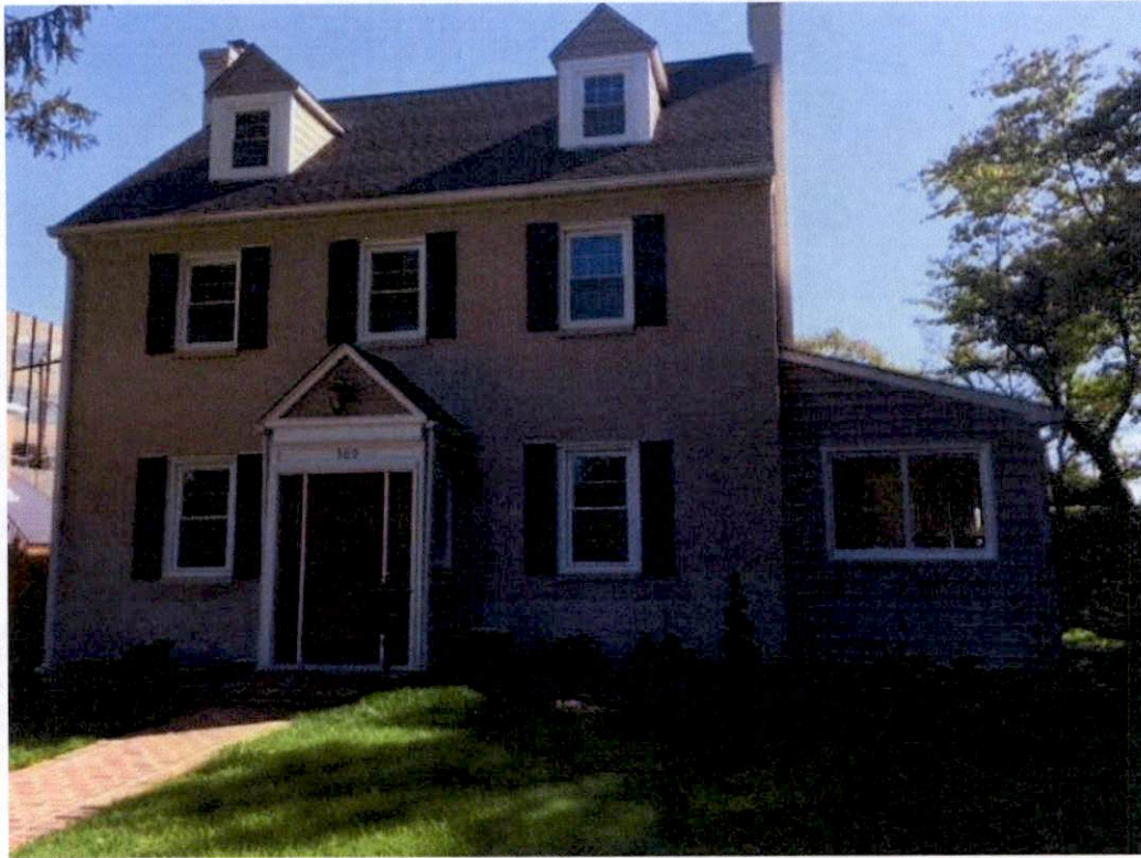
Front of residence, #309 W. Chesapeake Avenue, with existing addition on west building face.
