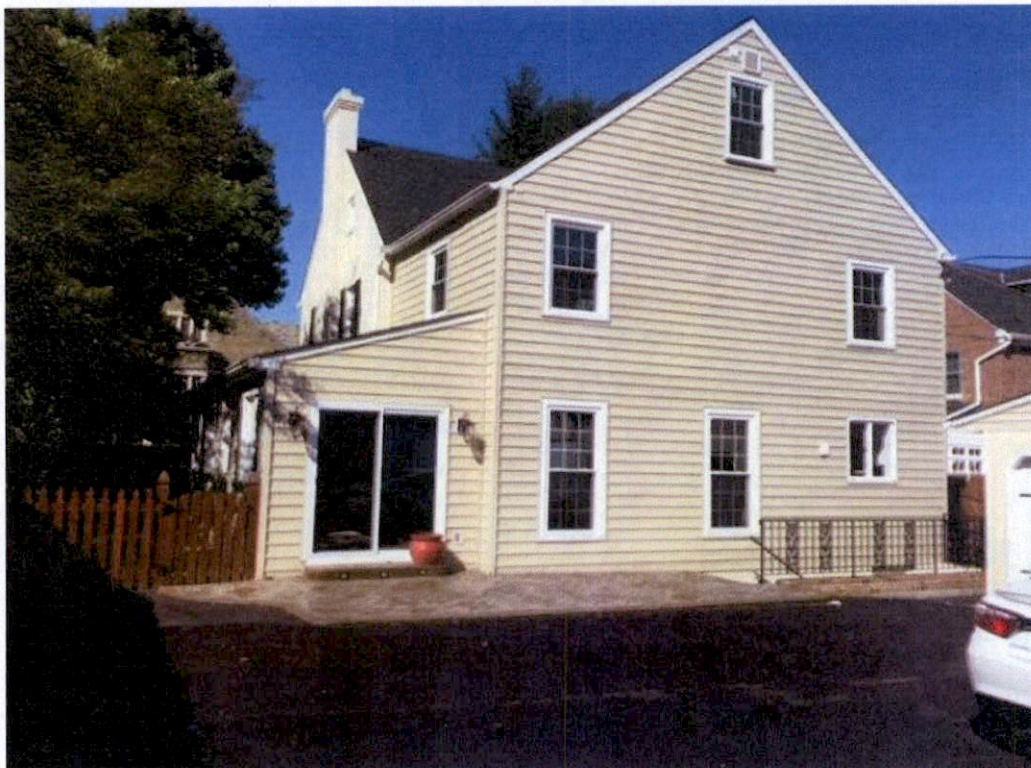
Rear of residence with existing addition on west building face and existing paved area.
