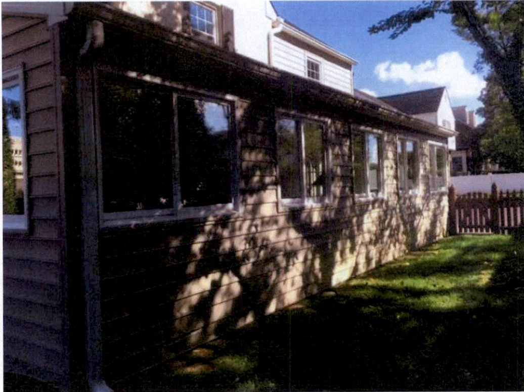
Existing addition on west building face.
