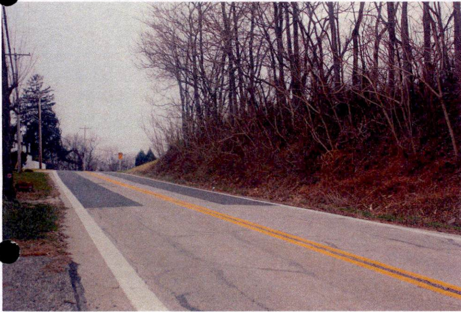
Facing west, site is to the right
