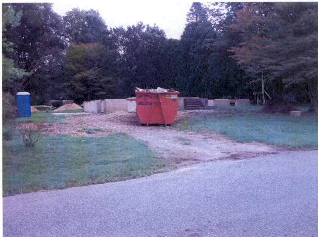
CONSTRUCTION AT 926 ELLENDALE DRIVE
