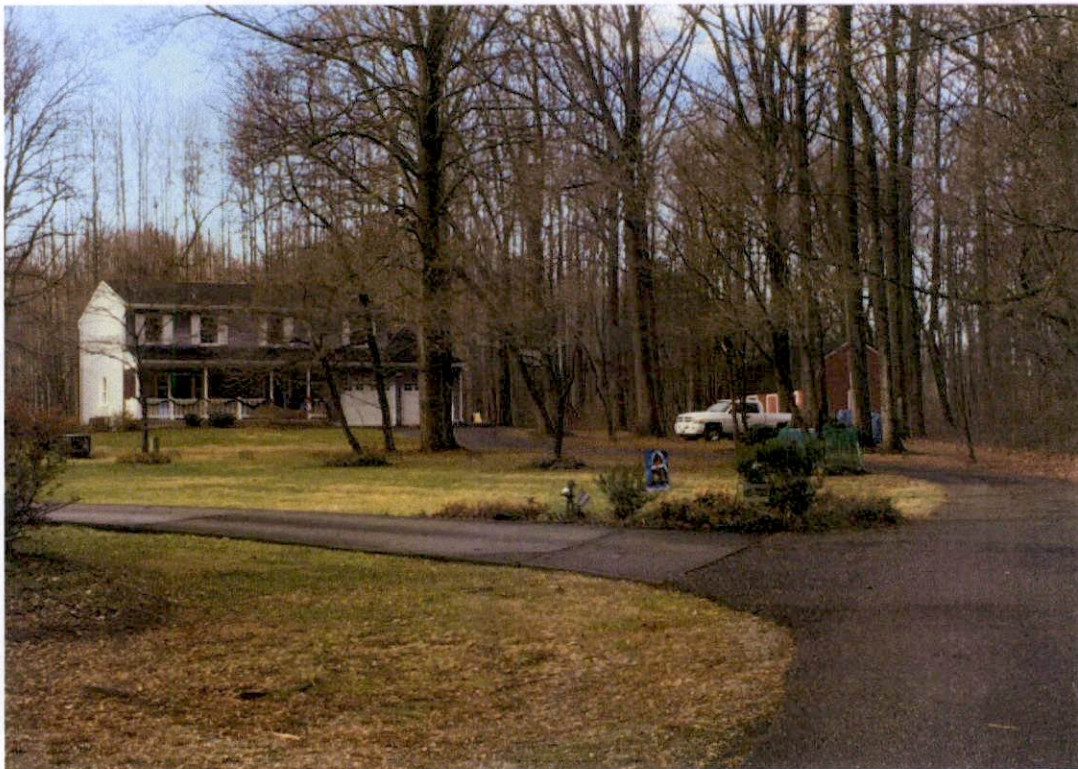
Front of adjacent dwelling, #12448 Jerusalem Road, and existing shed in front yard.
