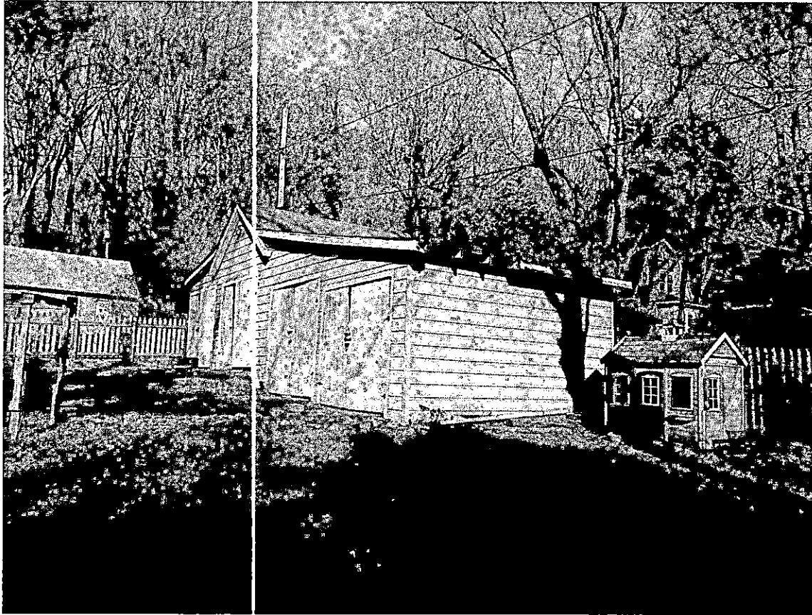
Side view of existing garage back yard.
