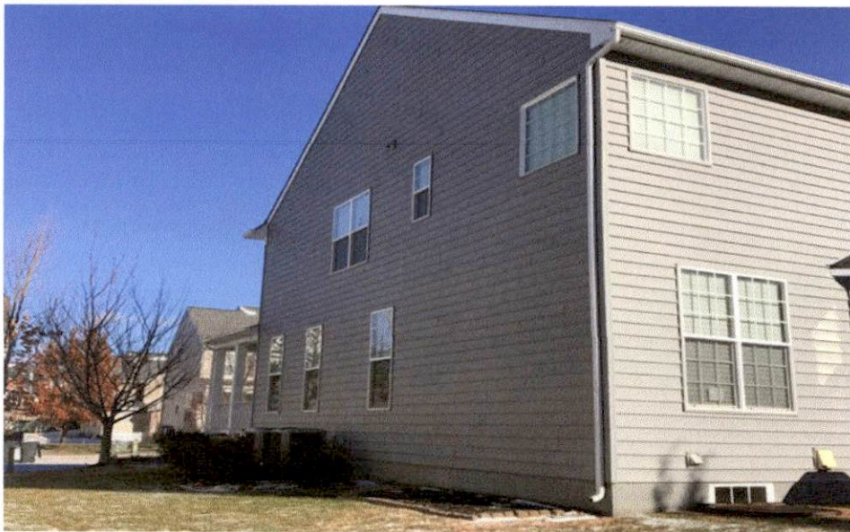
Left side Elevation – (picture taken from the rear)
